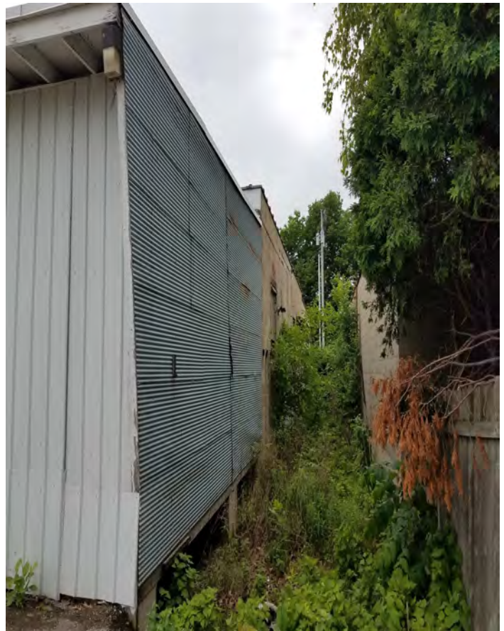
EXTERIOR OF NORTHEAST REAR OF RECEIVING AREA.
