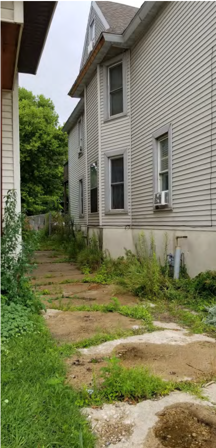
WEST SIDE OF APARTMENT.
