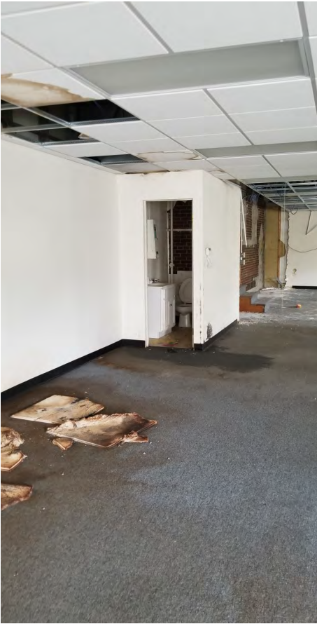
UPPER, MAIN SPACE FACING E WASHINGTON AVE.
