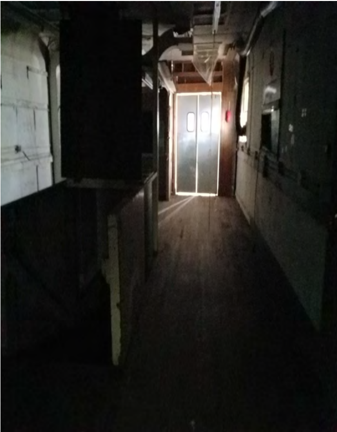
HALLWAY TO BASEMENT STAIRWAY (OPPOSITE REAR SPACE).
