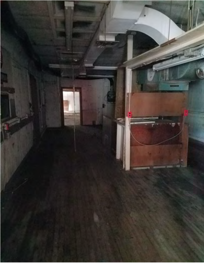
HALLWAY TO REAR SPACE (OPPOSITE BASEMENT STAIRWAY).
