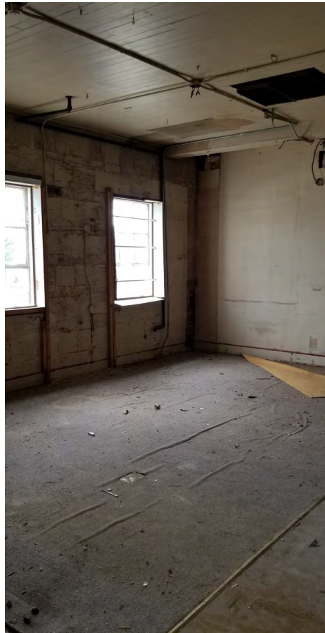
UPPER, TOP OF STAIRS #2.
