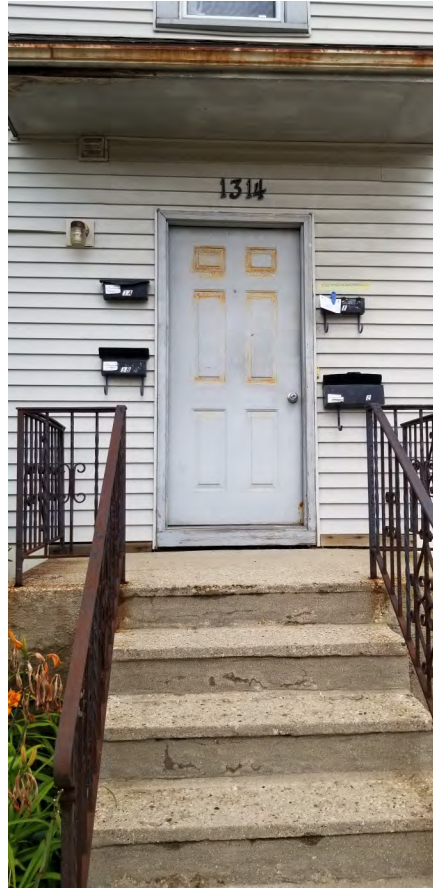
FRONT ENTRANCE, E WASHINGTON AVE.
