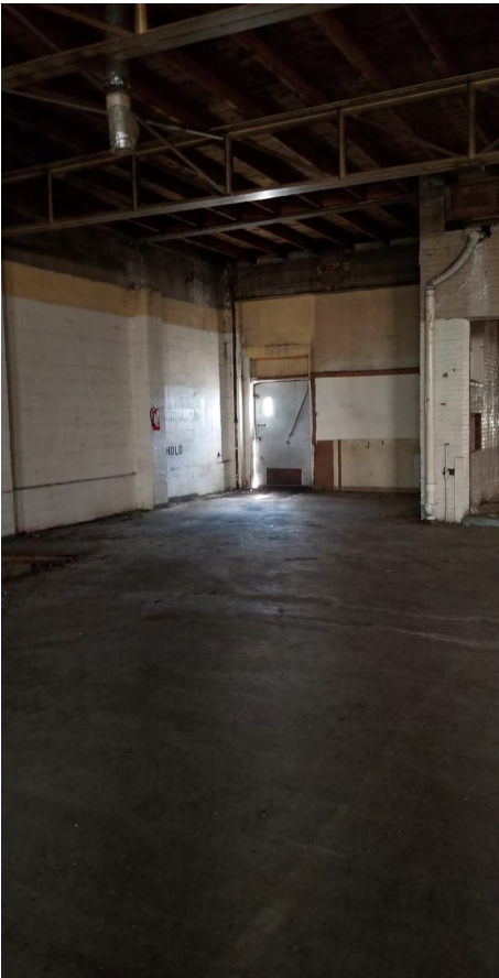
RECEIVING AREA, MAIN FLOOR.
