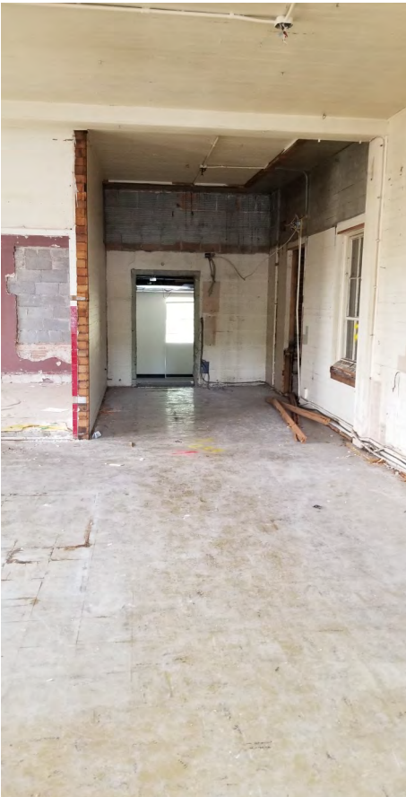
UPPER, TOP OF STAIRS #1.
