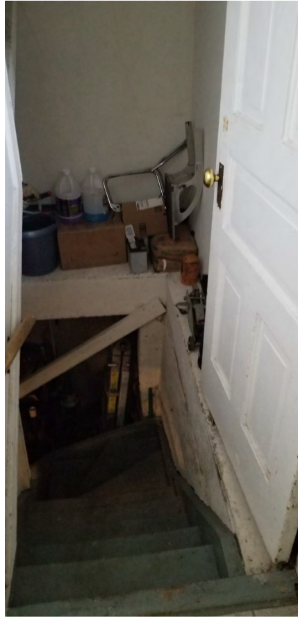
STAIRWAY TO BASEMENT.
