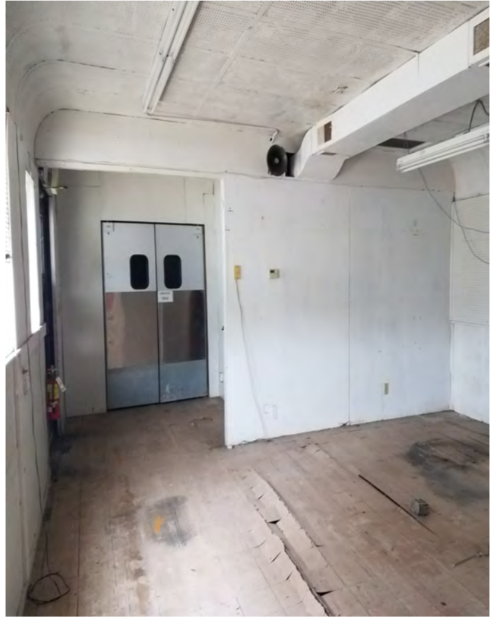
OPPOSITE OF FRONT ENTRANCE.
