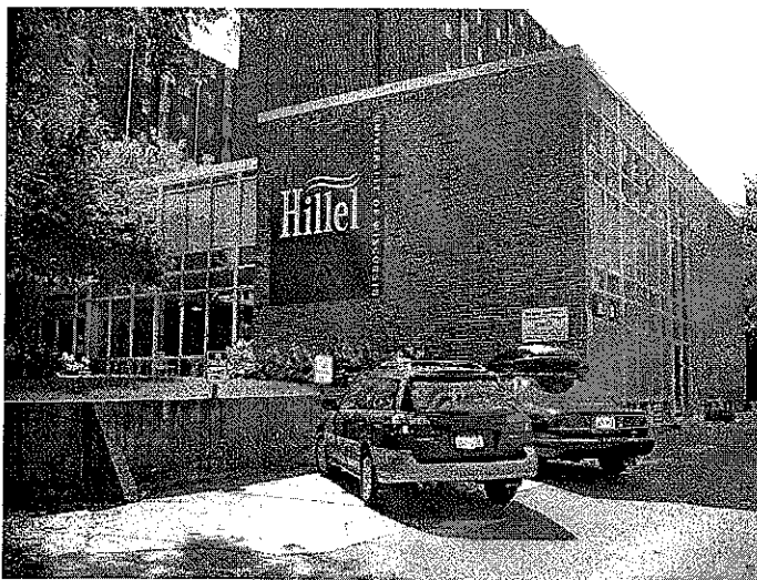
Figure 4. View From Alley Looking Towards The North Elevation
