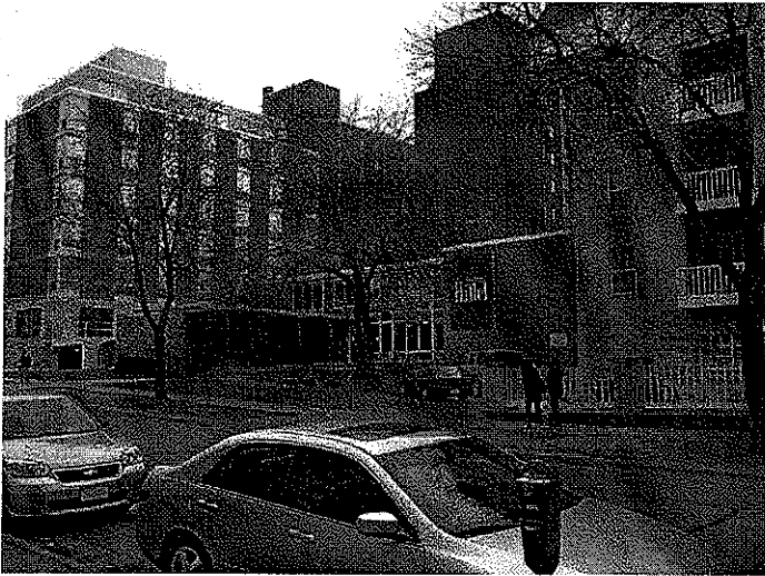
Figure 1. View From Langdon Looking Southeast
