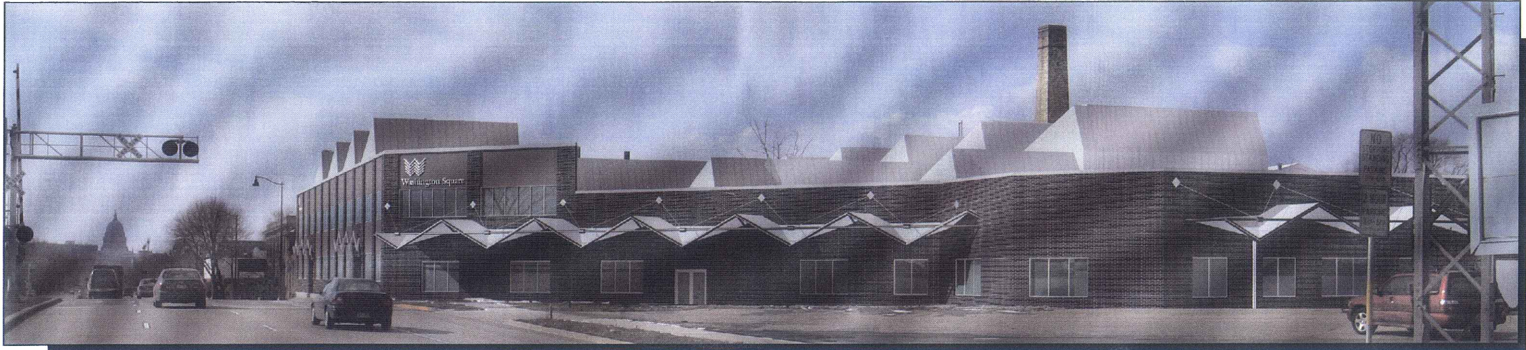
EAST ELEVATION (SOUTH PORTION) LOOKING DOWN EAST WASHINGTON
