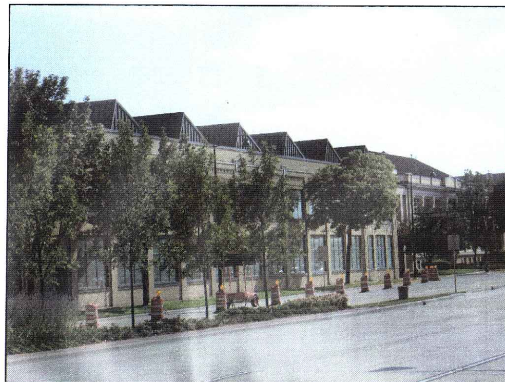
SOUTHWEST ADJACENT VIEW
