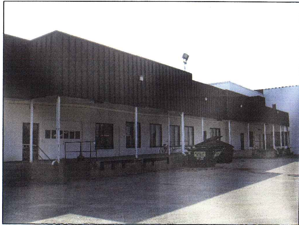
PARTIAL EAST ELEVATION - NORTH
