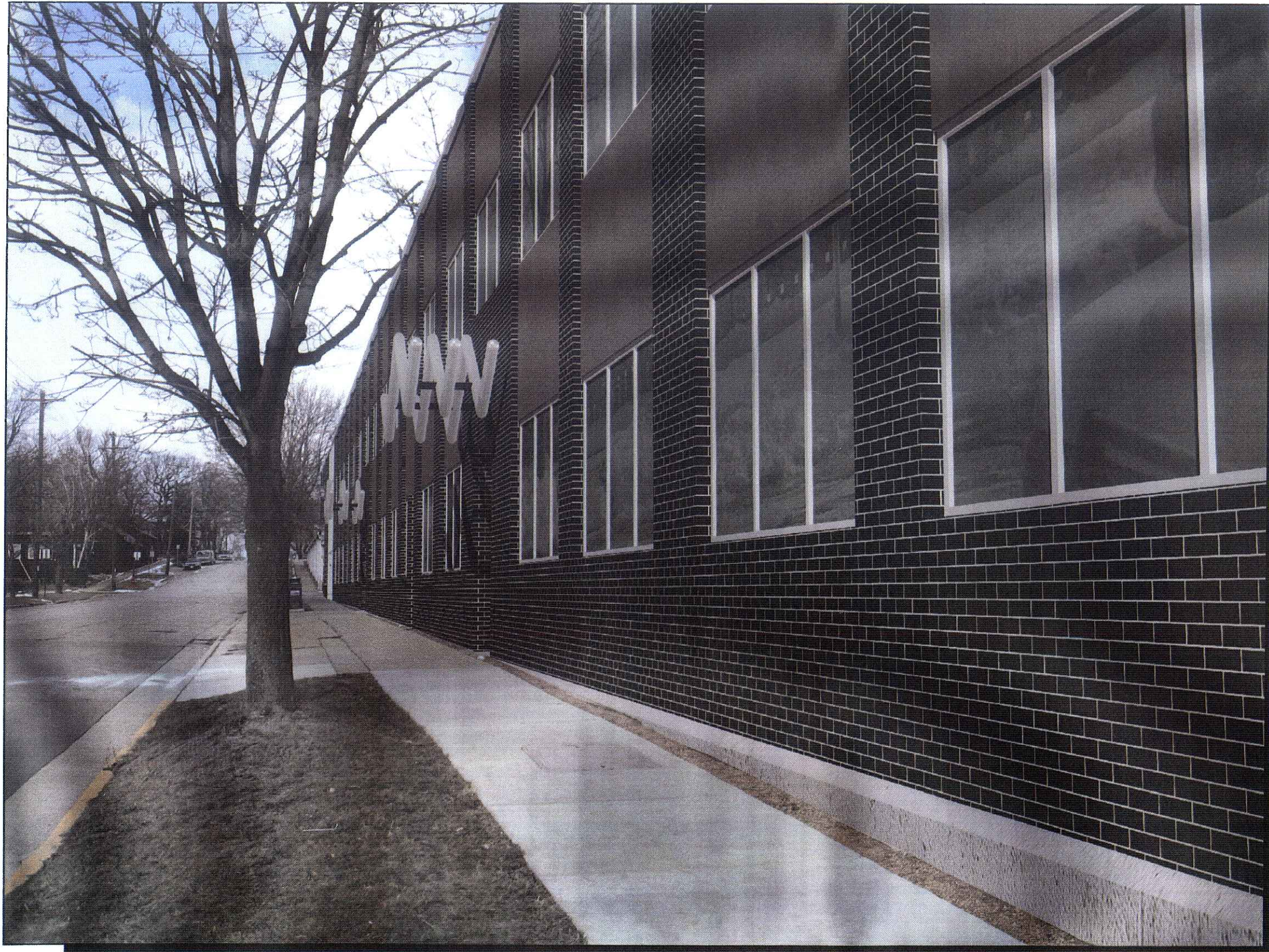
WEST ELEVATION OF NORTH DICKINSON STREET - SIDEWALK
