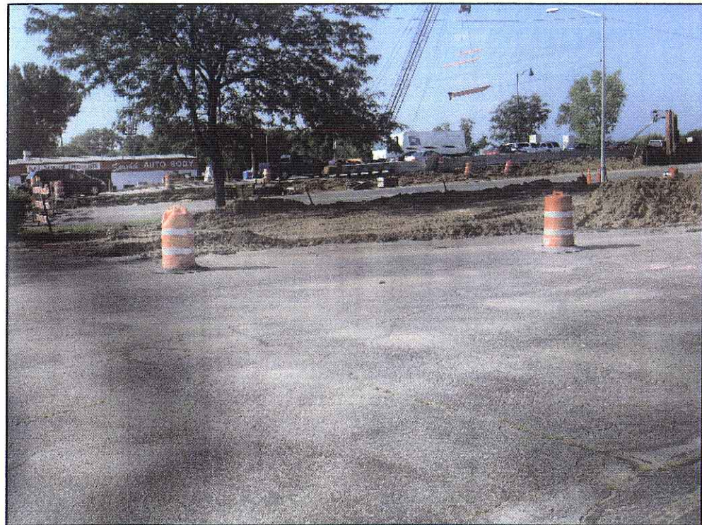
NORTHEAST ADJACENT VIEW
