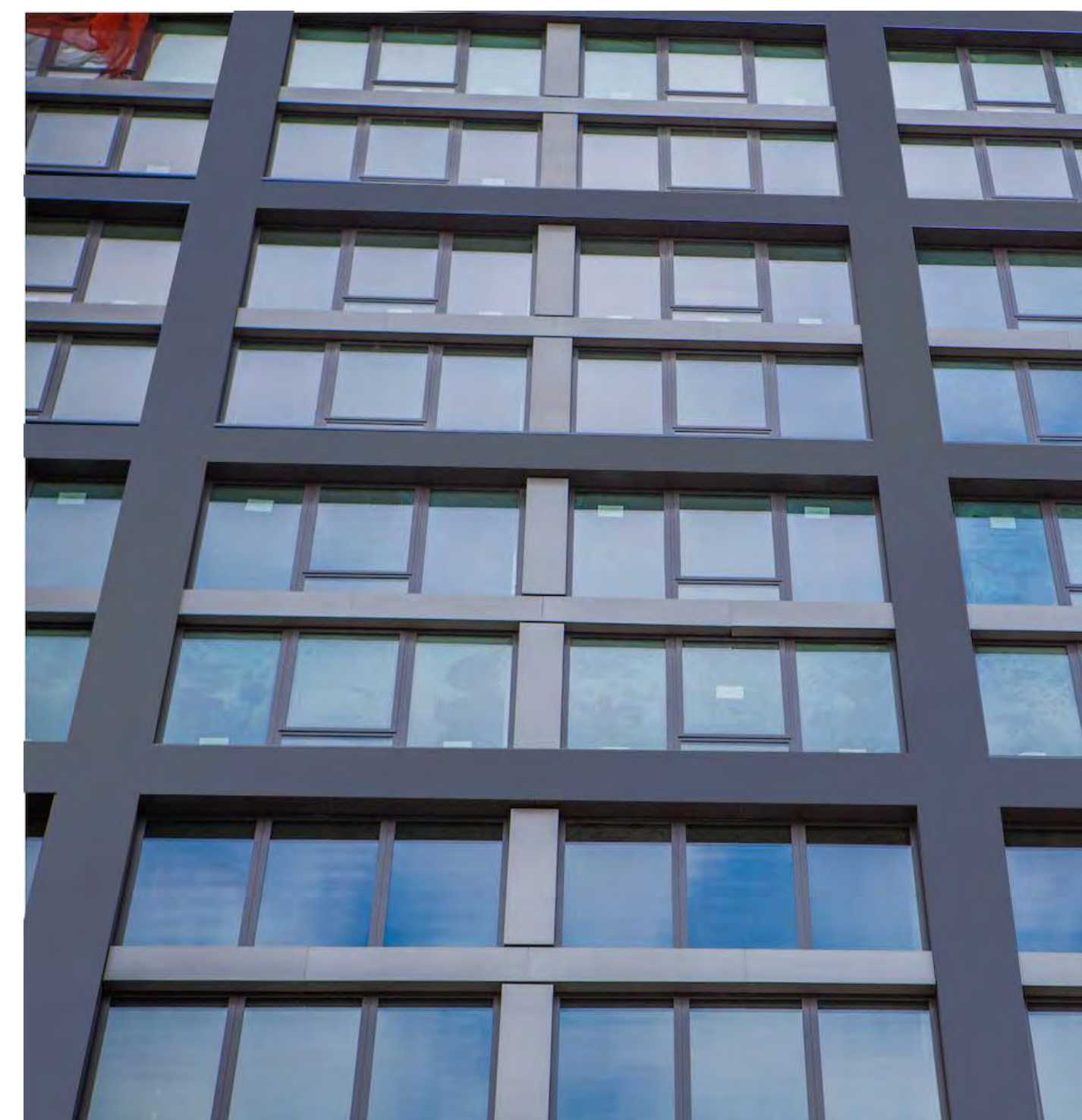
EWS-2 INSULATED METAL PANEL/ALUMINUM WINDOWS (SIM)
