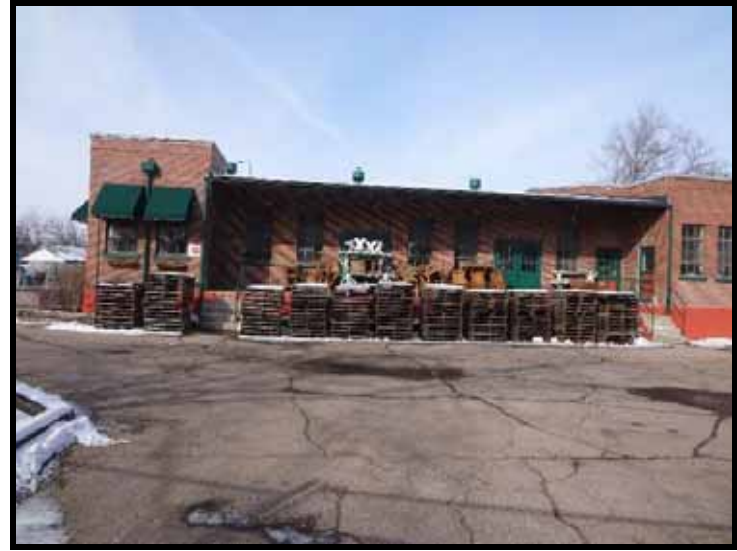
Existing One-Story Building (Proposed to Keep)
