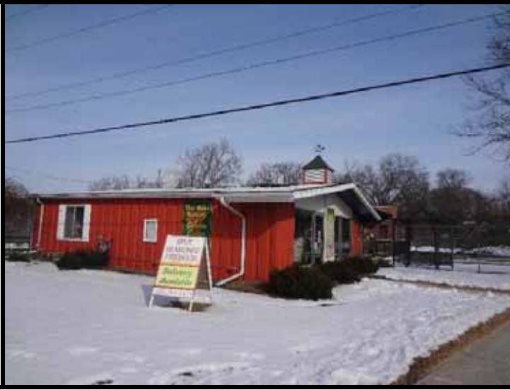
Existing One-Story Building on Site
