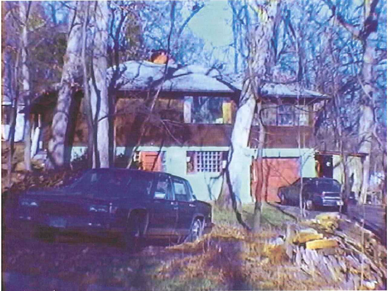
Demolition of existing house to construct a new single-story residence.
