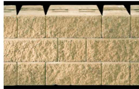
SAMPLE RETAINING WALL PATTERN & SCALE. SIMILAR STANDARD COLOR TO ONE SHOWN. ONCE MANUFACTURER IS SELECTED, SHOP DRAWINGS WILL BE REQUIRED FOR STANDARD INSTALLATION, COORDINATION WITH FENCE AND COLOR SAMPLES
