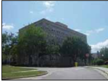
1 Langdon - Kennedy Manor Multi-Family Residential Stories – 6 Elevation 135.0 Feet (22 Feet Less than Project)
