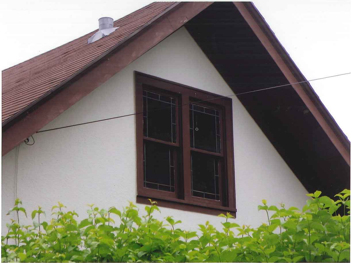
Existing Rear Window
