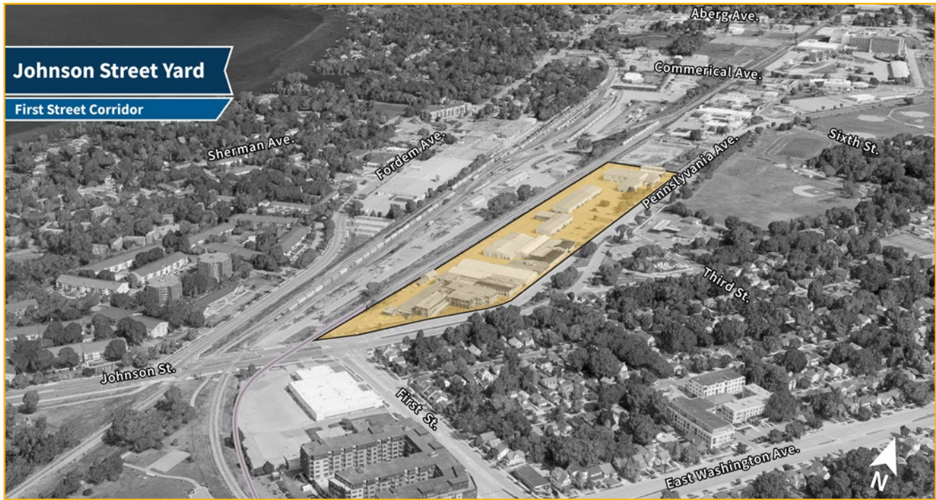
Figure 3.3: Johnson Street Yard Site Overview
