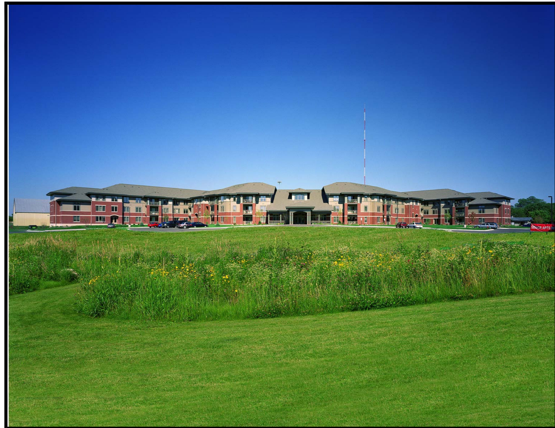
1 EXISTING PRAIRIE PARK SENIOR APARTMENTS NORTH-EAST OF SITE SCALE: NOT TO SCALE
