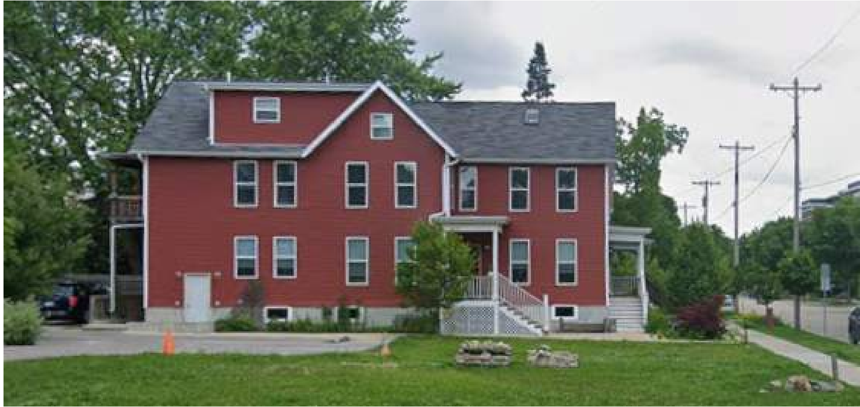
710-712 E DAYTON STREET AS PART OF THE PD TEXT, 710-12 E DAYTON STREET (EXISTING VINYL FACADE) TO GET RE-CLAD WITH ENGINEERED WOOD.
