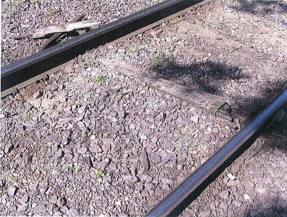
Between Corry and Winnebago Broken Tie June 6, 2005
