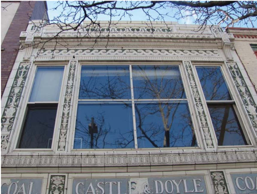
Figure 7. The central second floor window is a non-original assembly consisting of painted 2x wood framing supporting four panes of glass and a separate, similarly divided storm window.
