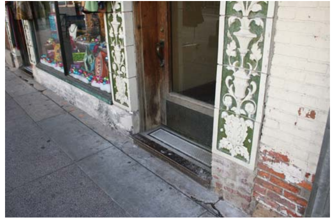
Exterior: View of existing stoop to second floor access
