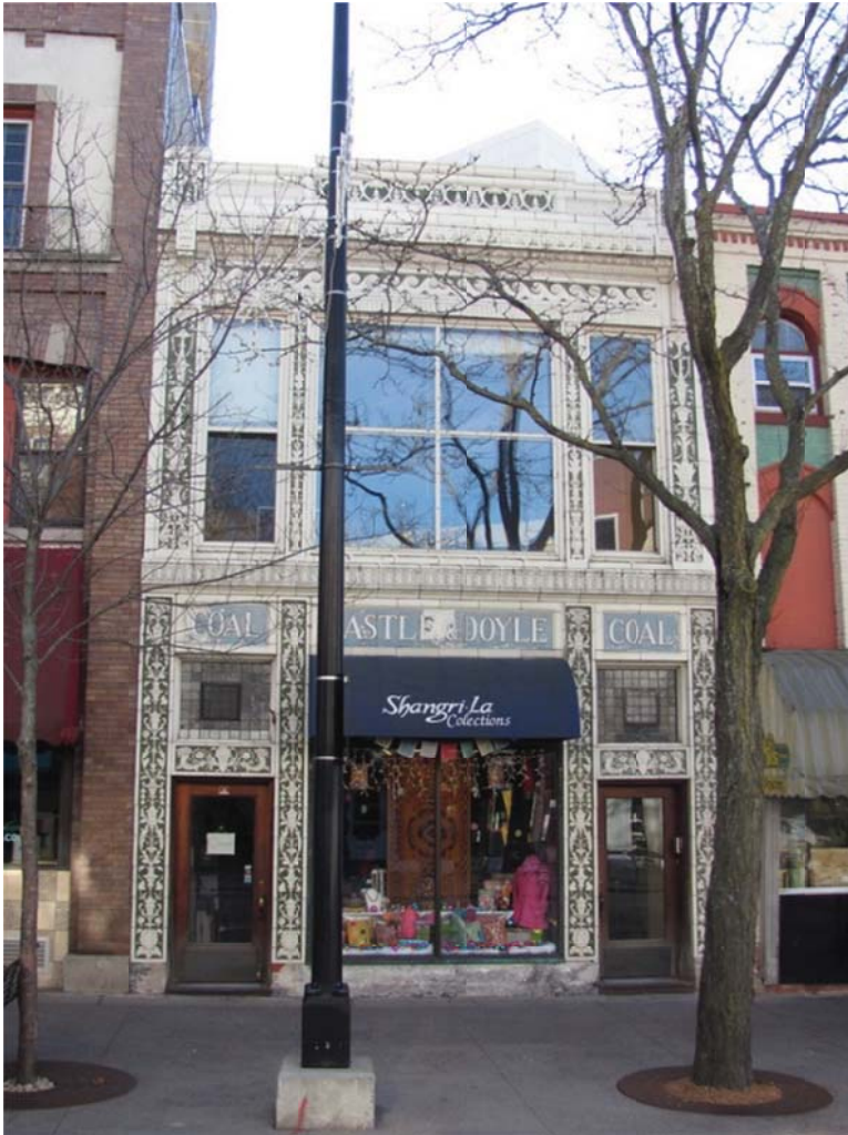
Figure 1. Overall view of the State Street facade.
