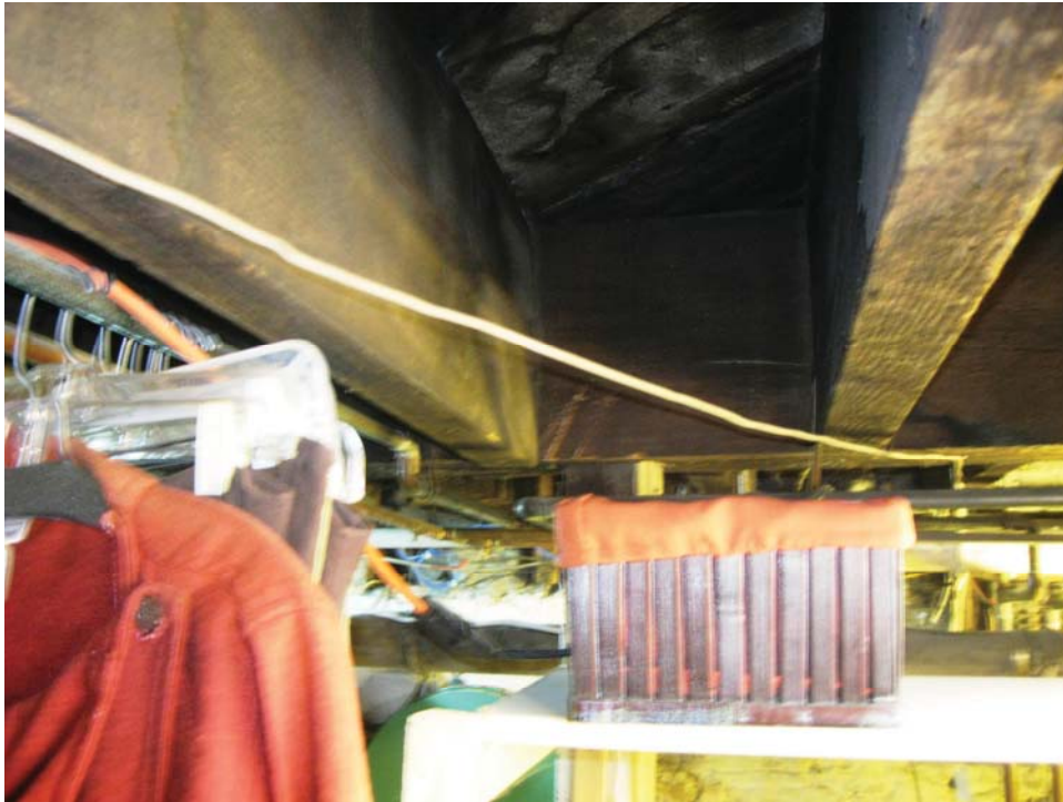
Photo 5 – 1 st floor joist framing
