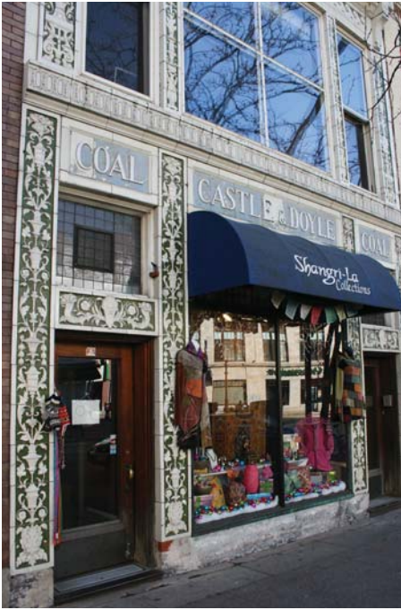
View of Front Facade
