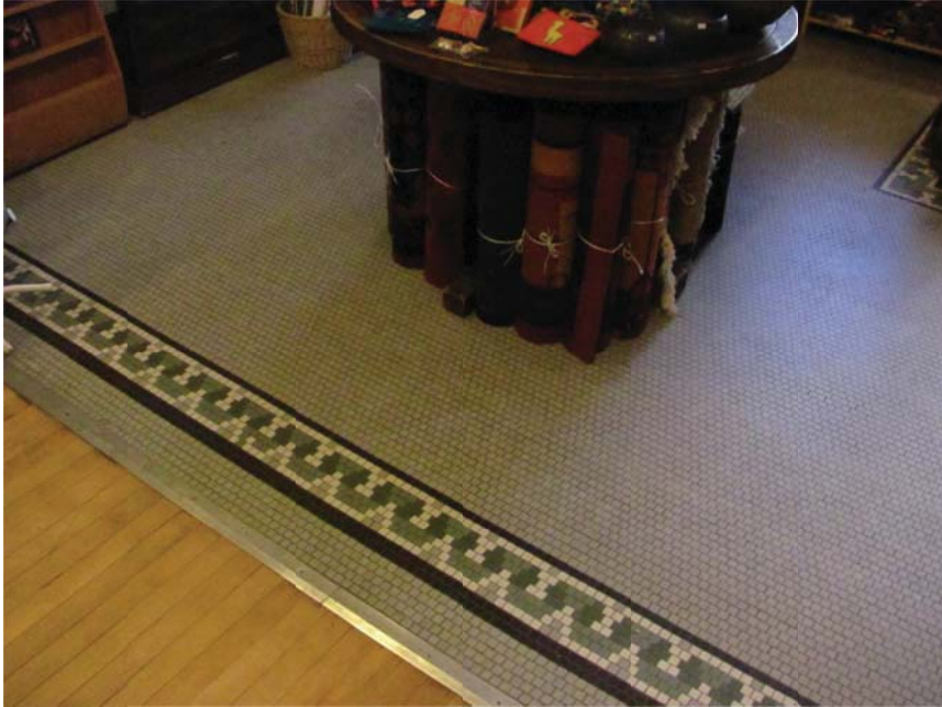
Figure 15. Hardwood and mosaic ceramic tile flooring in the first floor retail space.
