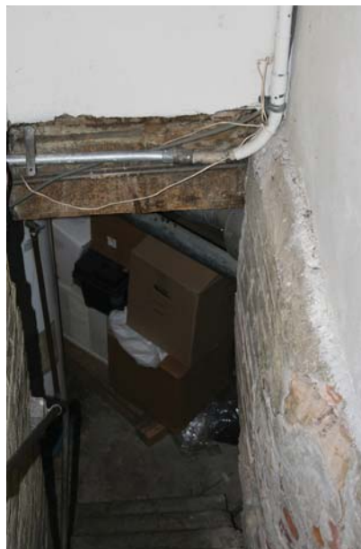
Basement Access Stair
