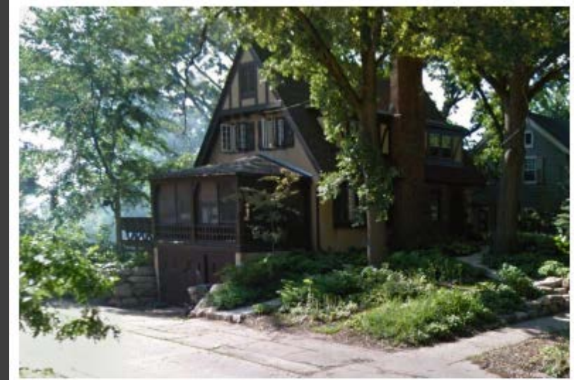
114 BASCOM PI - DEMONSTRATES SHED DORMER ON STEEP SLOPE OF SECOND LEVEL ROOF TO PROVIDE HABITABLE SPACE UNDER THE ROOFLINE
