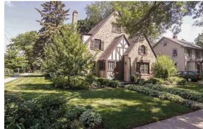
2314 VAN HISE - DEMONSTRATES SHED DORMER ON STEEP SLOPE OF SECOND LEVEL ROOF TO PROVIDE HABITABLE SPACE UNDER THE ROOFLINE
