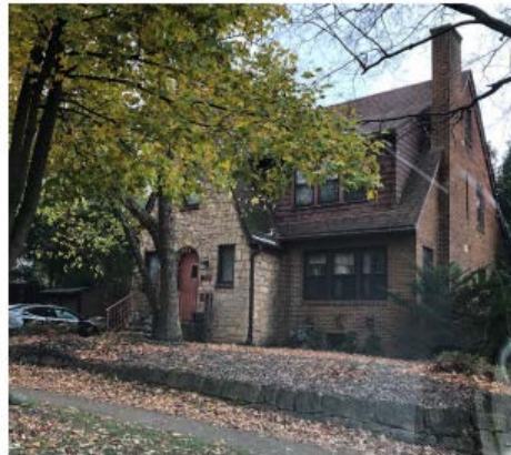
122 N. ALLEN ST - DEMONSTRATES SHED DORMER ON STEEP SLOPE OF SECOND LEVEL ROOF TO PROVIDE HABITABLE SPACE UNDER THE ROOFLINE. DORMER IS CLAD IN WOOD MATERIAL.
