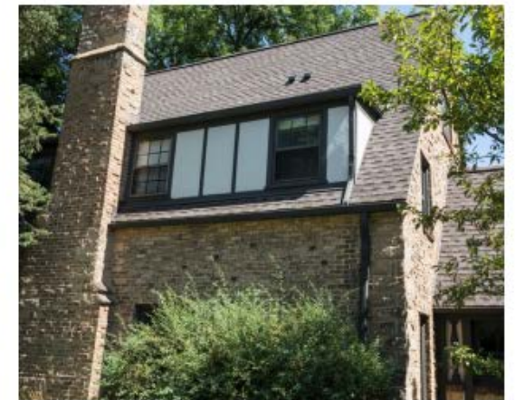
2314 VAN HISE - DEMONSTRATES SHED DORMER ON STEEP SLOPE OF SECOND LEVEL ROOF TO PROVIDE HABITABLE SPACE UNDER THE ROOFLINE
