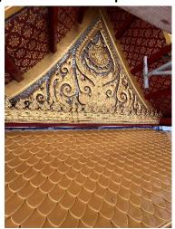
Phase two is in full swing with the Royal Thai Pavilion. This phase includes cleaning the biologicals off the structure, painting, replacing the gold leaf where needed, and replacing the glass mosaic tiles. This phase is expected to finish in fall 2024.
