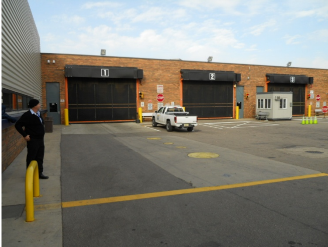
Figure 33: Entrance Door 3, Exit Door 4
