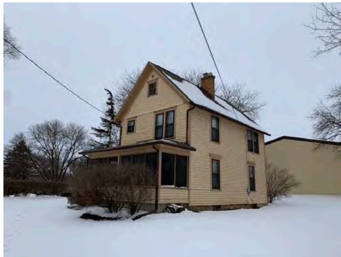
701 McCormick – Exterior view from SE
