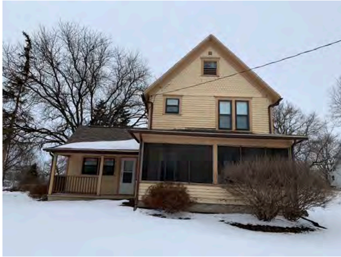
701 McCormick – Exterior view from South
