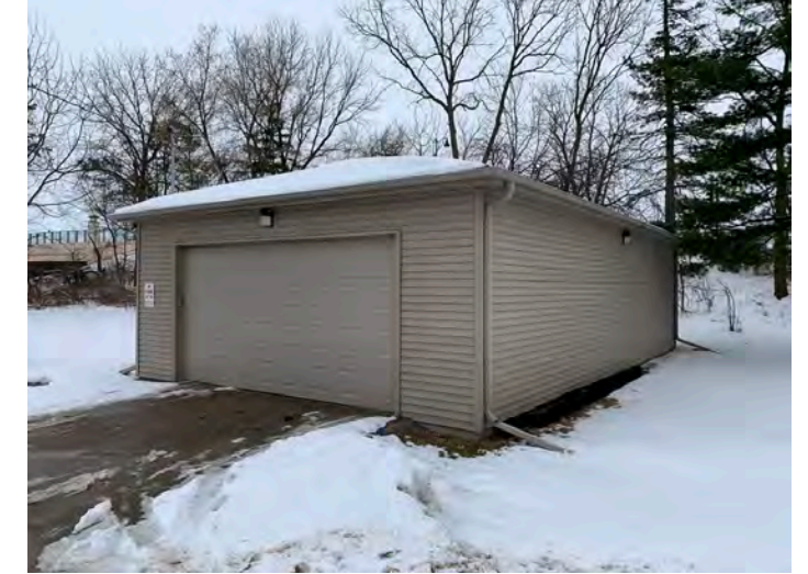
3046 Commercial – Garage from West
