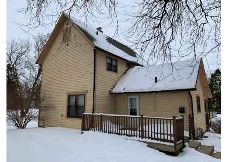
701 McCormick – Exterior view from NW
