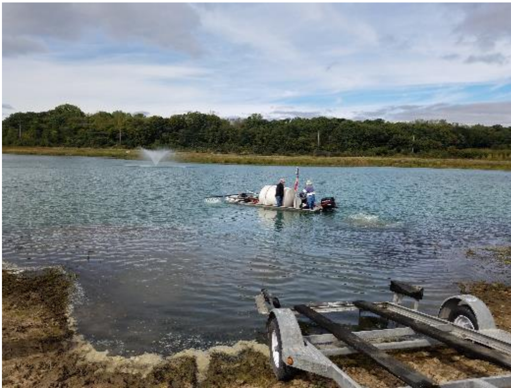
Figure 17. Coagulant application at Autumn Lake, Madison, WI.
