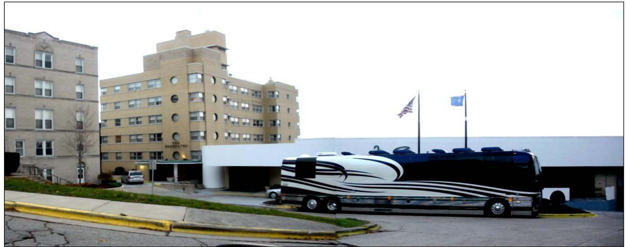
Slope is 10%, Maximum Allowed by Code is 5%
