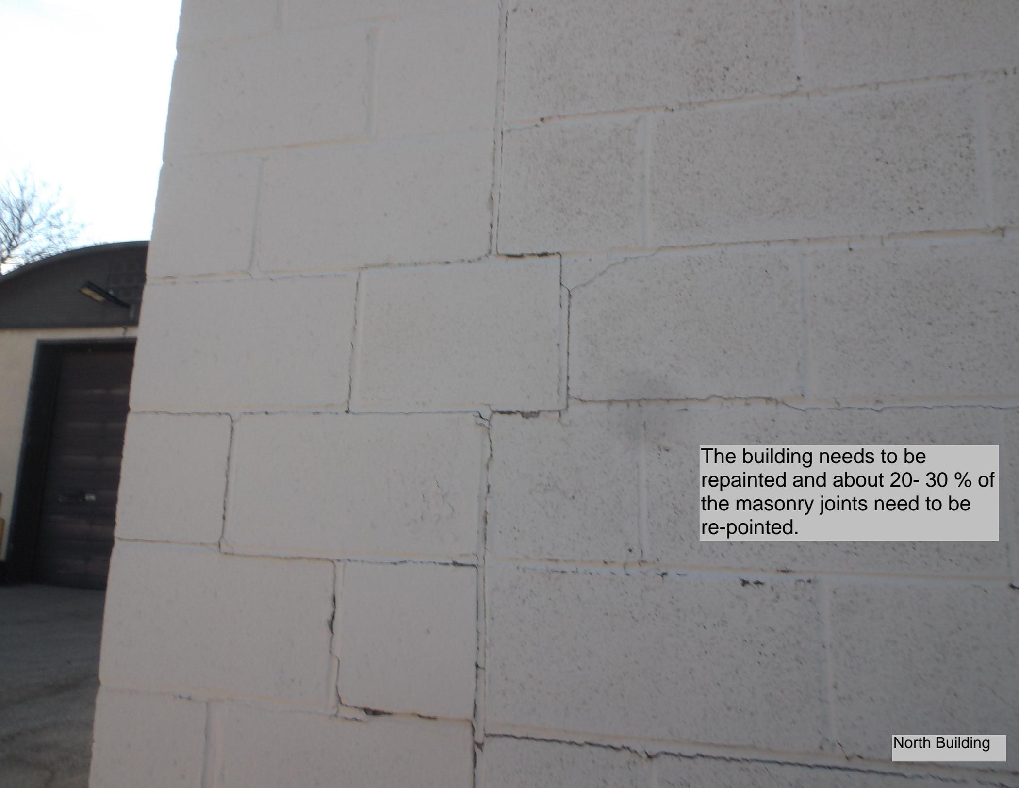
The building needs to be repainted and about 20- 30 % of the masonry joints need to be re-pointed.
