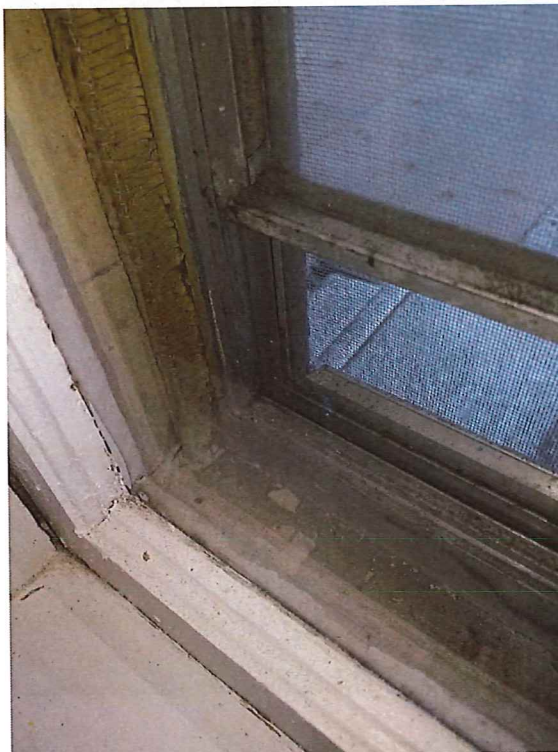
Window 9 1 st floor Pantry Lower sash opens about 2 inches, missing storm window
