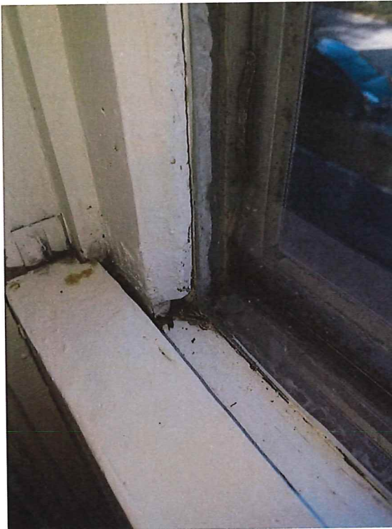
Window 13, 14 Front Bedroom 2 nd story Sash rot, missing counter weights, broken sash, missing and broken storm windows
