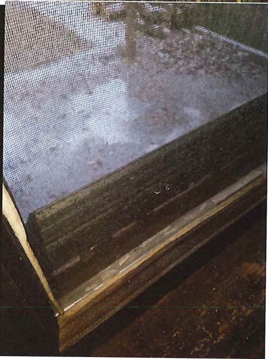
Window 8 1 st floor South in addition Broken glass, missing storm window, twisted frame
