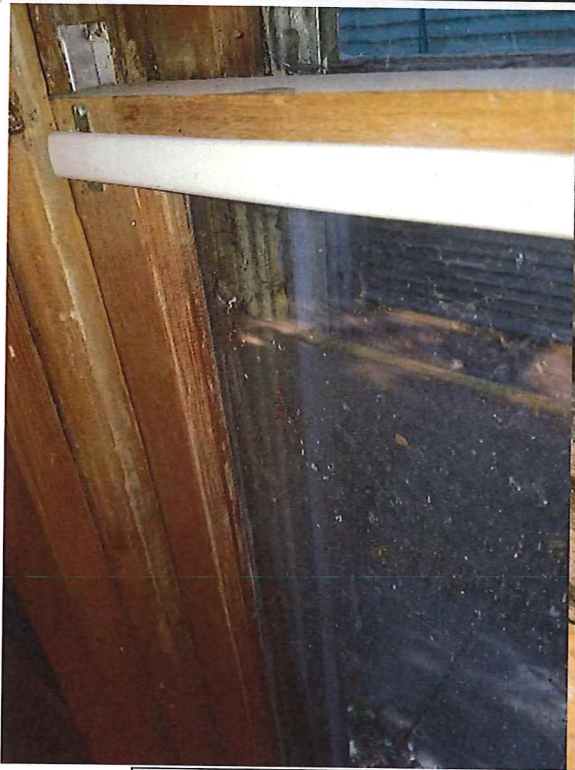
Window 5, 6 1 st floor Sash rot from exposed wood and condensation, missing counter weights, missing storm windows, alignment off
