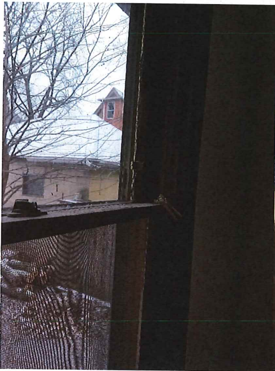
Window 8 1 st floor South in addition Broken glass, missing storm window, twisted frame
