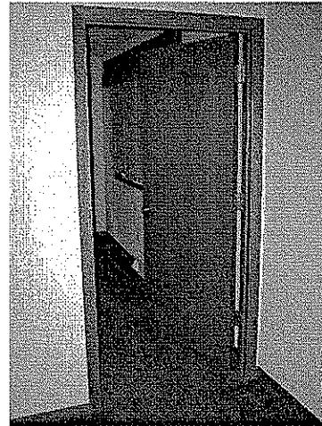
Wood Doors Condition - Varies Quantity: 14 Pre- Hung; 2 Bi-Fold; 2 Hollow Metal
