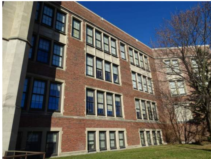
4. VIEW OF ORIGINAL CLASSROOM WING
