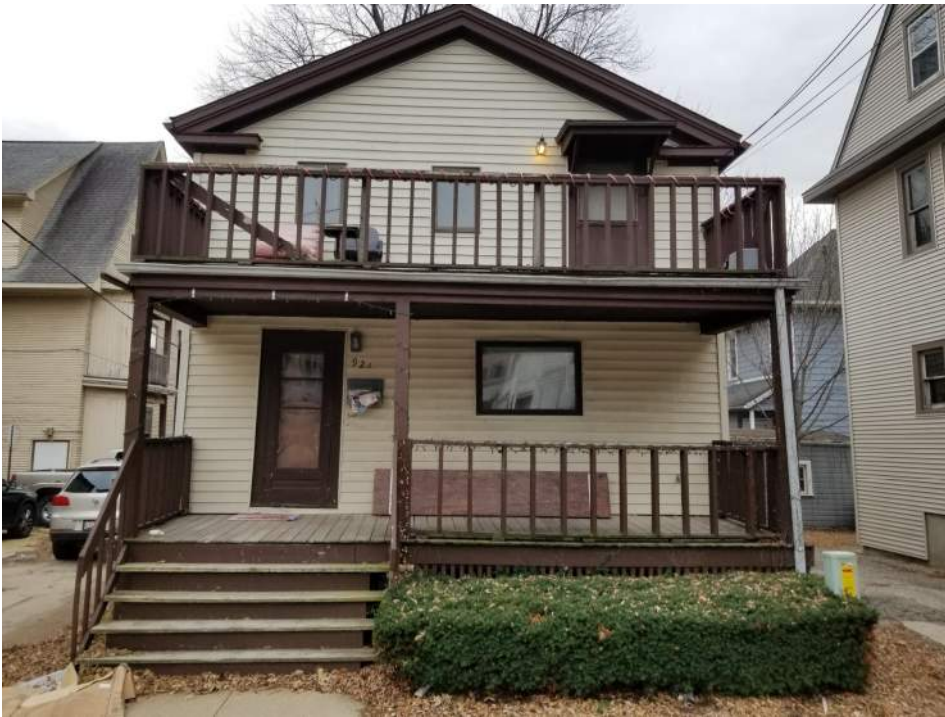
Figure 2. North elevation of 923 Clymer. Original materials have been replaced or covered with vinyl siding and windows infilled. The porch has been rebuilt.
