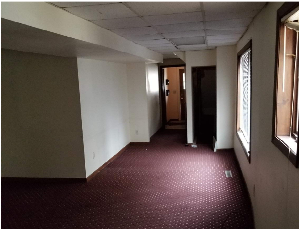
Figure 8. First floor living room.
