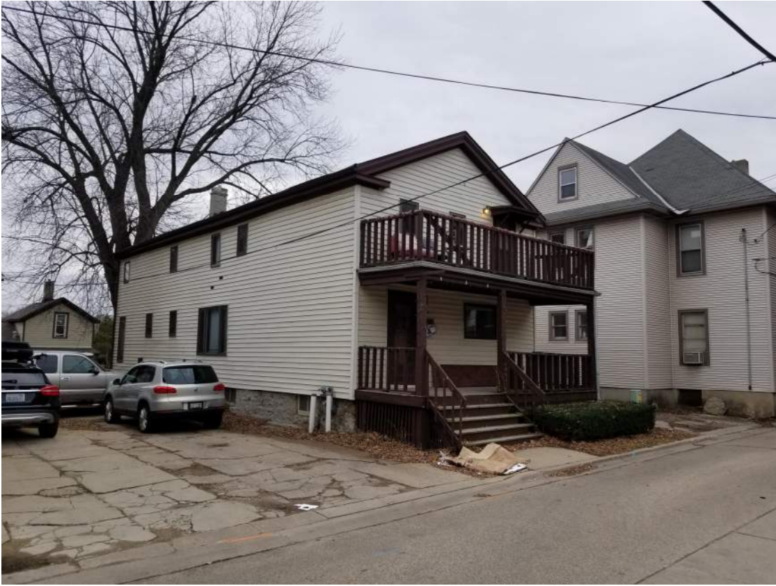
Figure 1. North east corner of the building.
