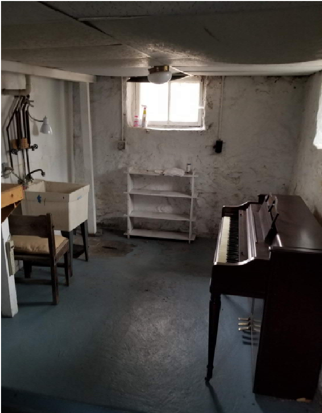
Figure 4. Basement Utility Room.
