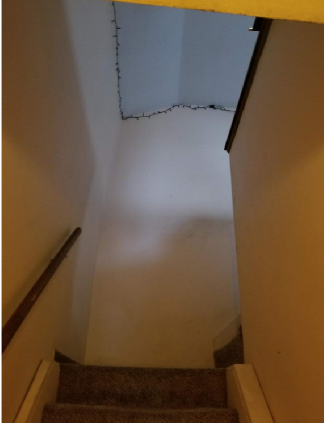
Figure 7. Primary stair to second floor.
