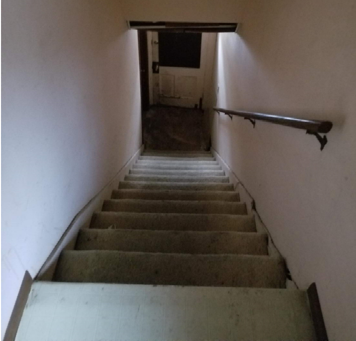
Figure 5. Basement access stairs.
