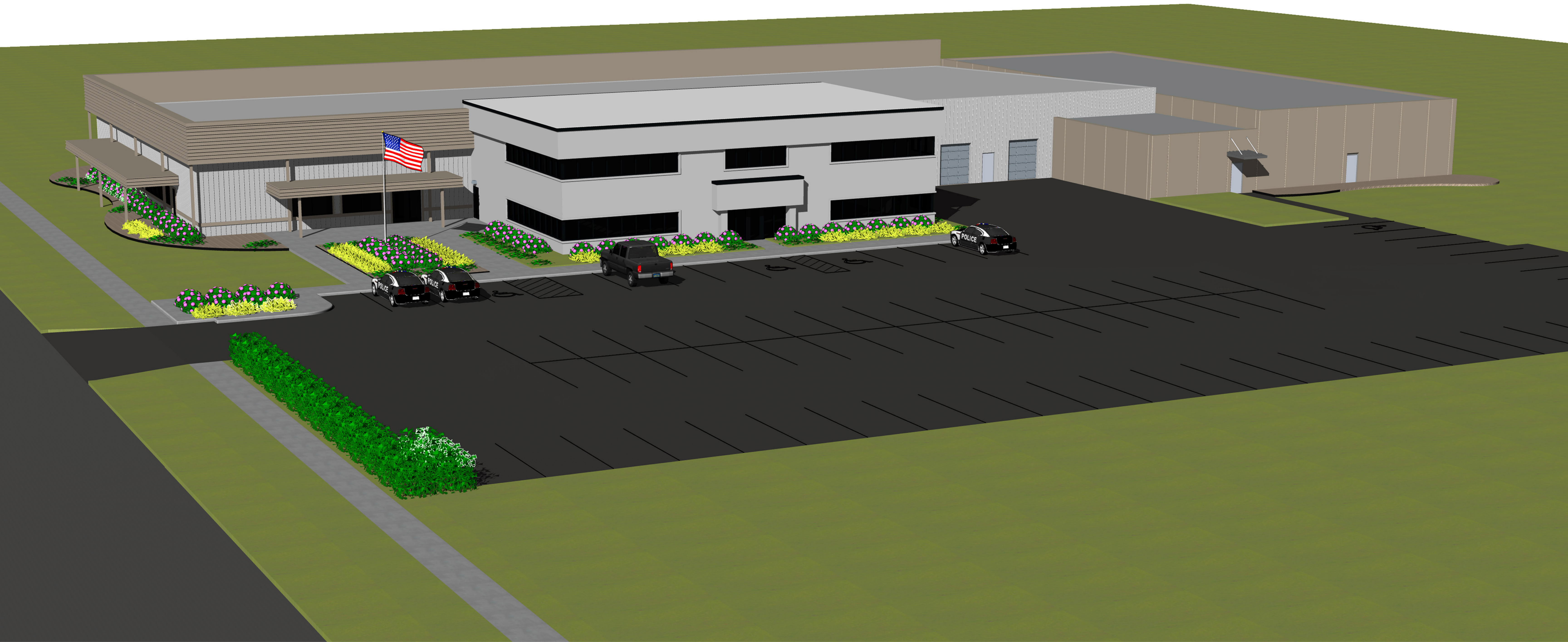
Madison Police Training Facility
