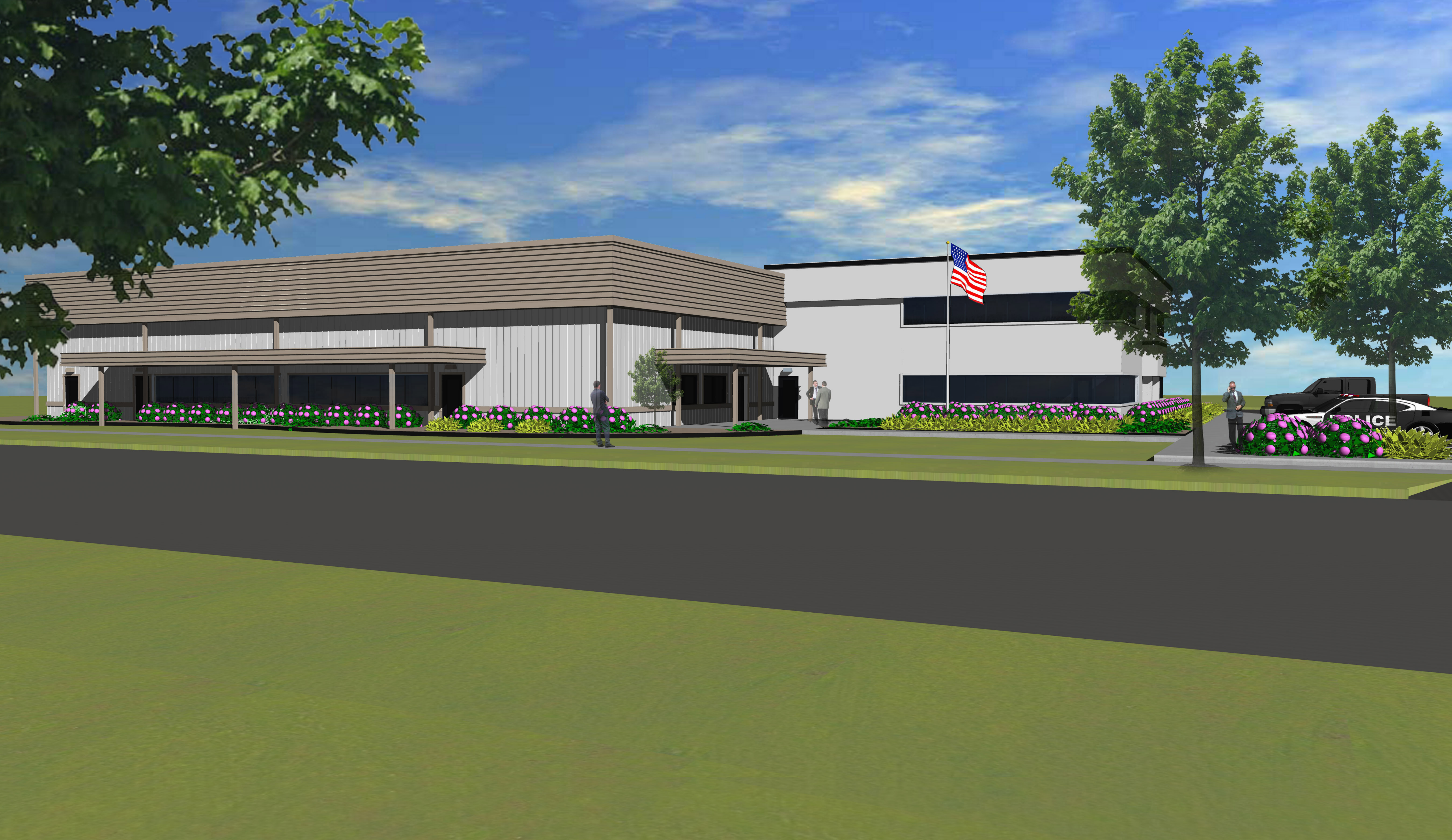
Madison Police Training Facility
