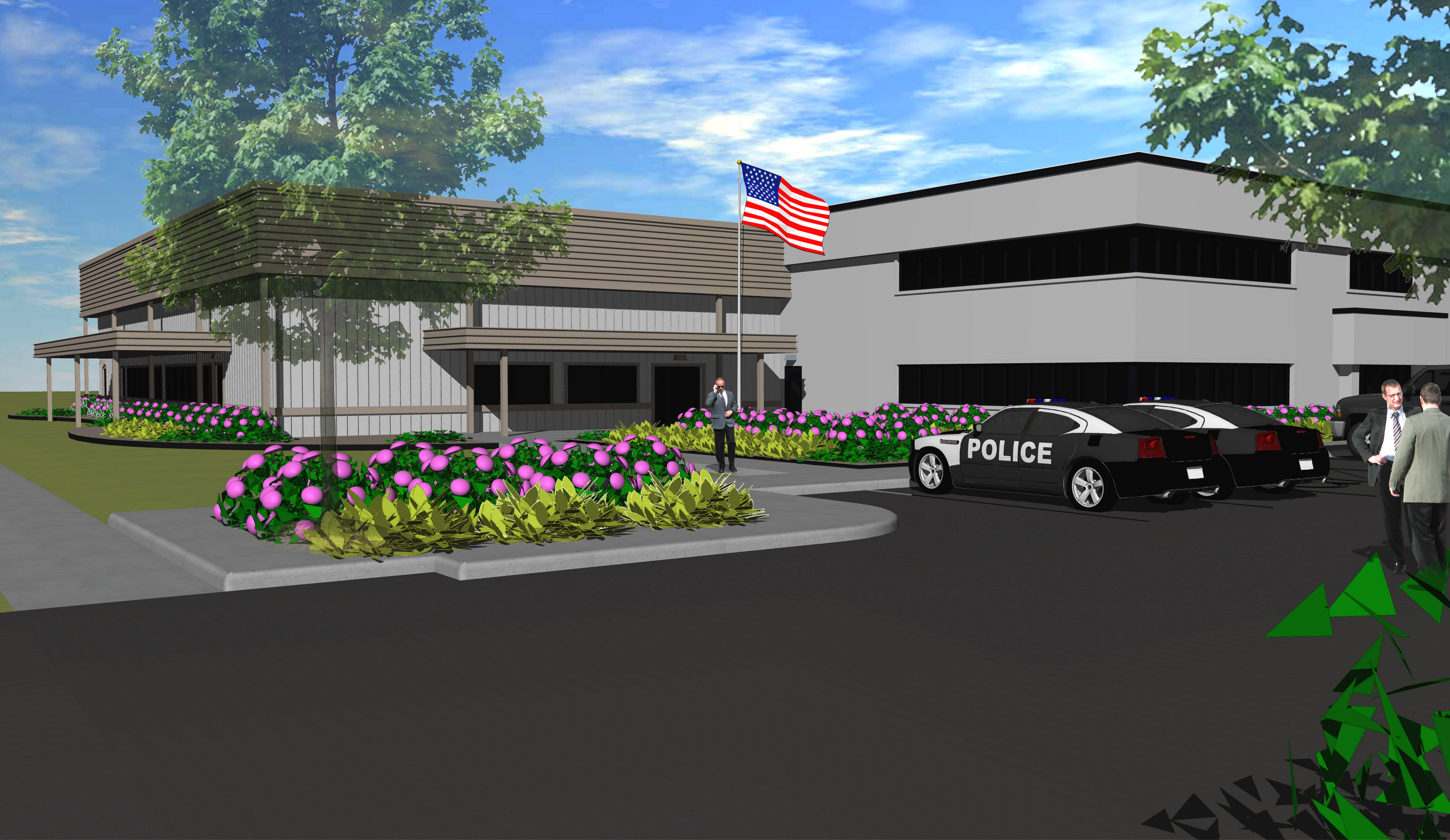
Madison Police Training Facility
