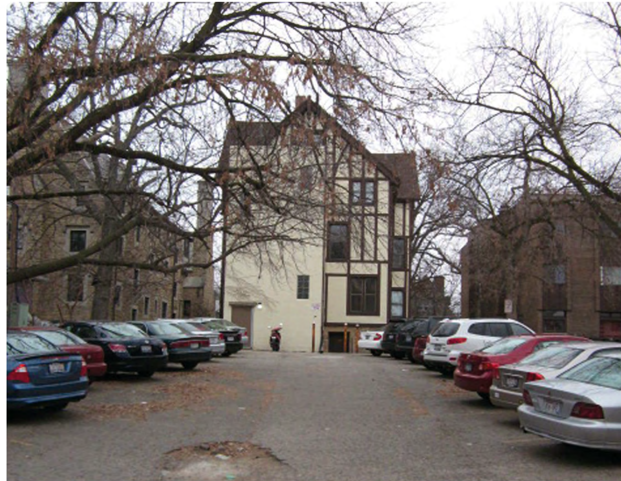
210 Langdon Street - Rear Elevation
