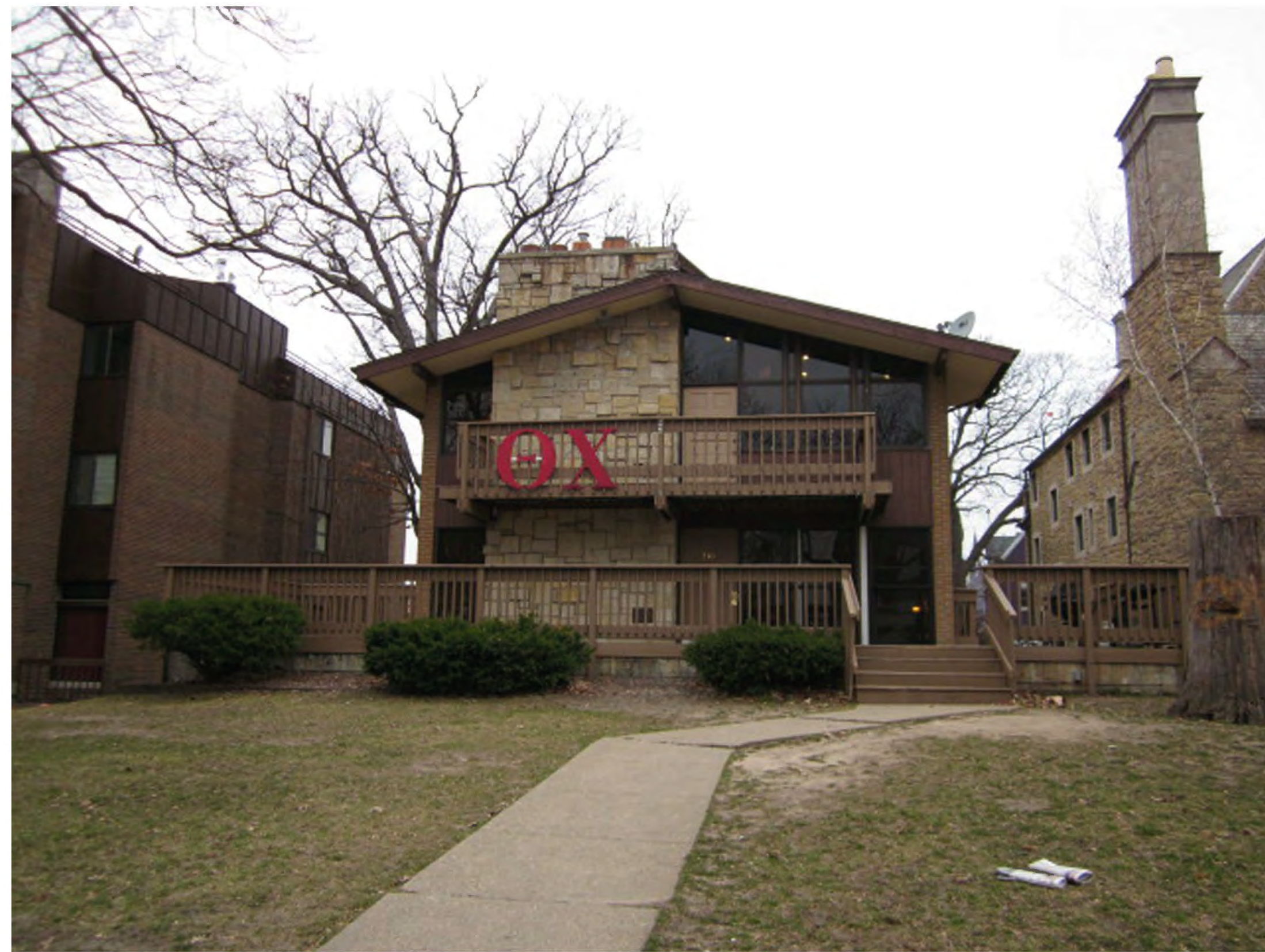
210 Langdon Street-Langdon Elevation
