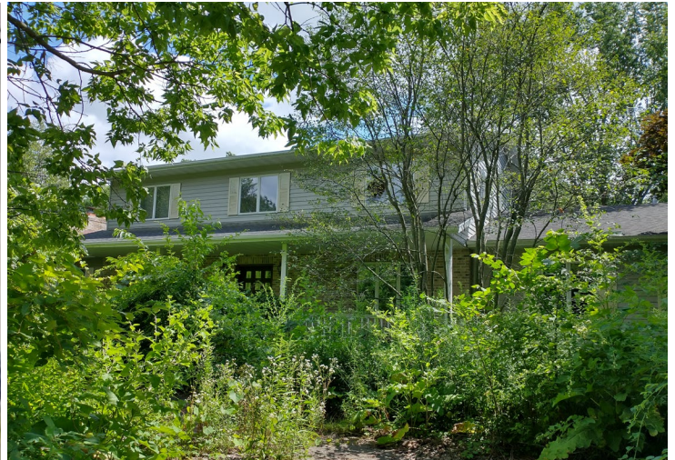
Photo from City of Madison Building Inspection
