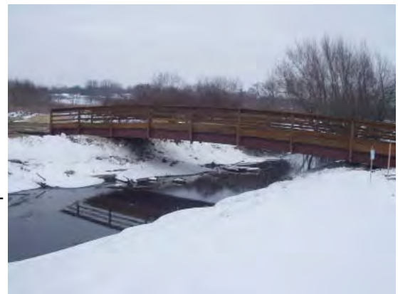
Photo: Bridge in Nine Springs E-Way near Baxter Park, joint County and City project, photo courtesy of Dane County Parks
