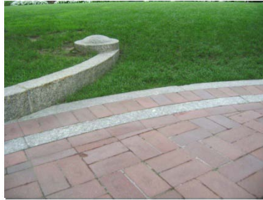
4 Lawn with Granite Curb and Brick Paving with Granite Trim Details SCALE: NTS
