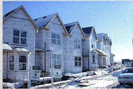
Townhouses in Grandview Commons during construction
