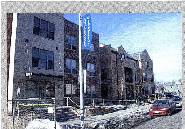
The Renaissance mixed-use buildings on the 800 block of Williamson Street also incorporated a historic structure in their Redevelopment Proposal.
