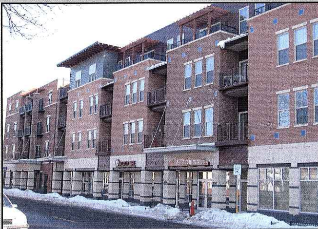
Kennedy Place, a four story mixed-use development on Atwood Avenue.
