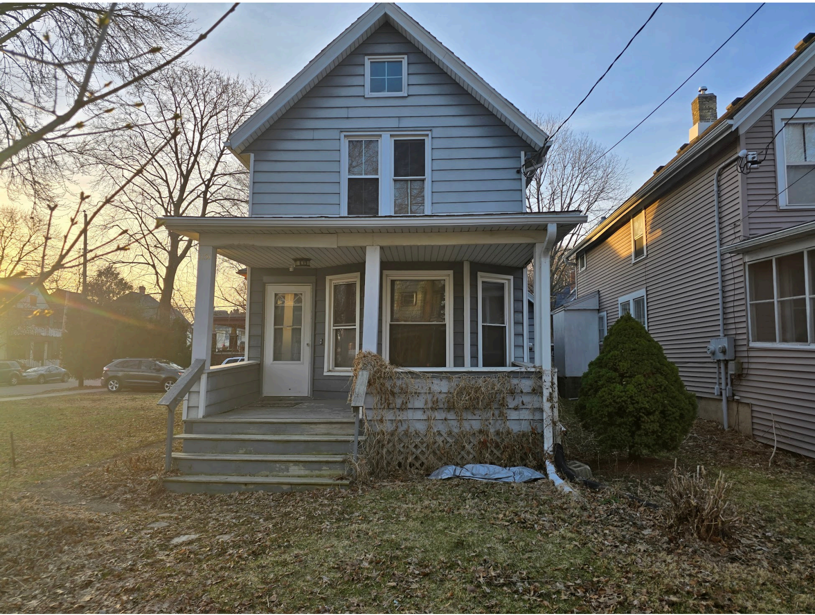
Front elevation of the existing single-family residence at 1151 Jenifer Street, which will remain on one of the proposed lots.
