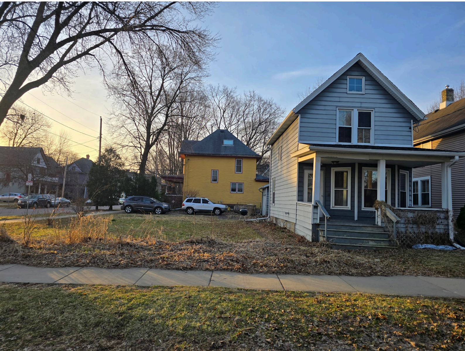
Subject property at 1151 Jenifer Street showing the existing single-family residence and side yard area where the proposed lot division will occur.
