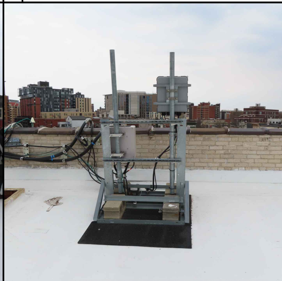
E EXISTING EQUIPMENT SLED MOUNT
