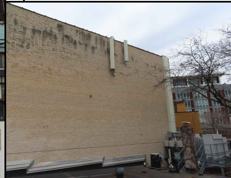
E U.S. CELLULAR GAMMA SECTOR ANTENNAS
