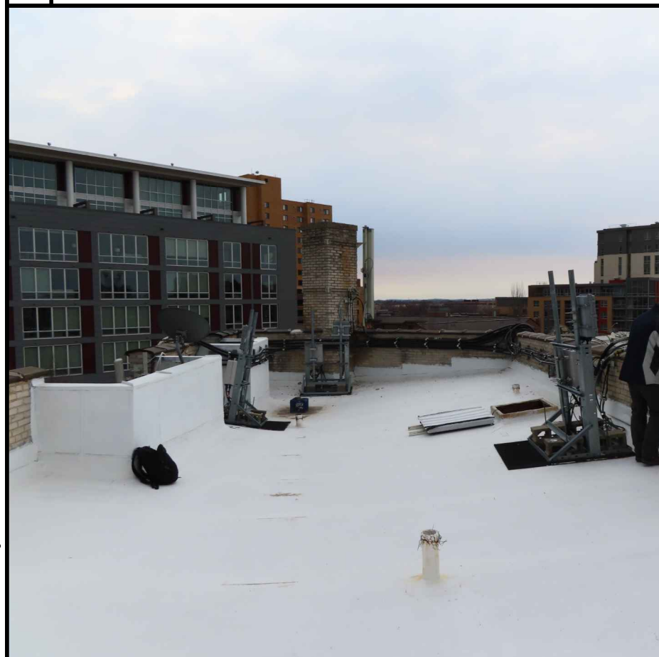
D EXISTING ROOFTOP OVERVIEW
