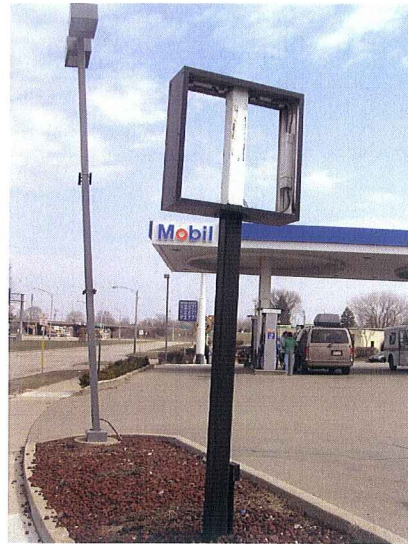
Broken Sign, Leaning Light Post 4601 Verona Rd March 30, 2006
