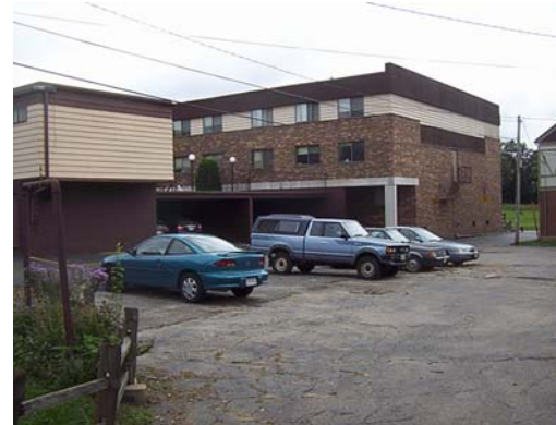
View from back of Knickerbocker Place looking Towards existing multifamily bldg and park.
