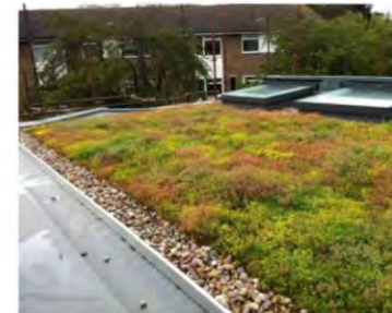
FULL SUN SEDUM CARPET GREEN ROOF WITH BALLAST EDGING - SEE PLANTING PLAN FOR MORE INFORMATION
