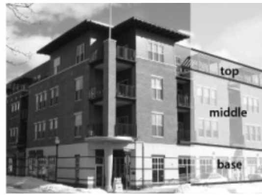
Figure D7: Building Articulation
