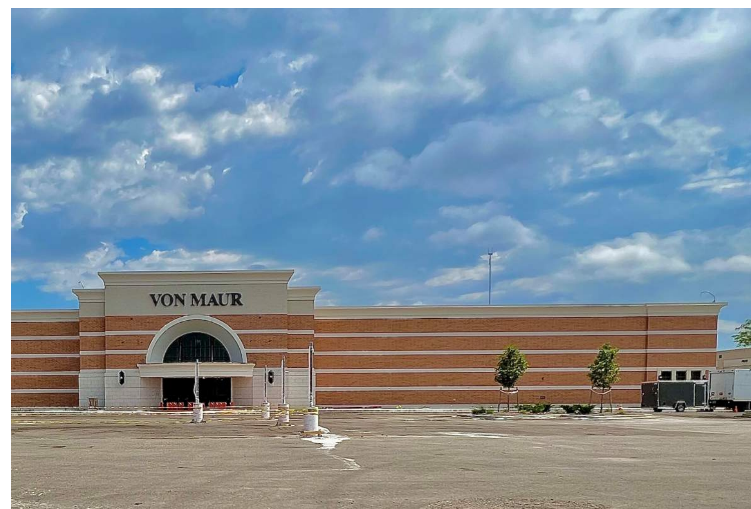
VON MAUR WEST EXTERIOR WALL
