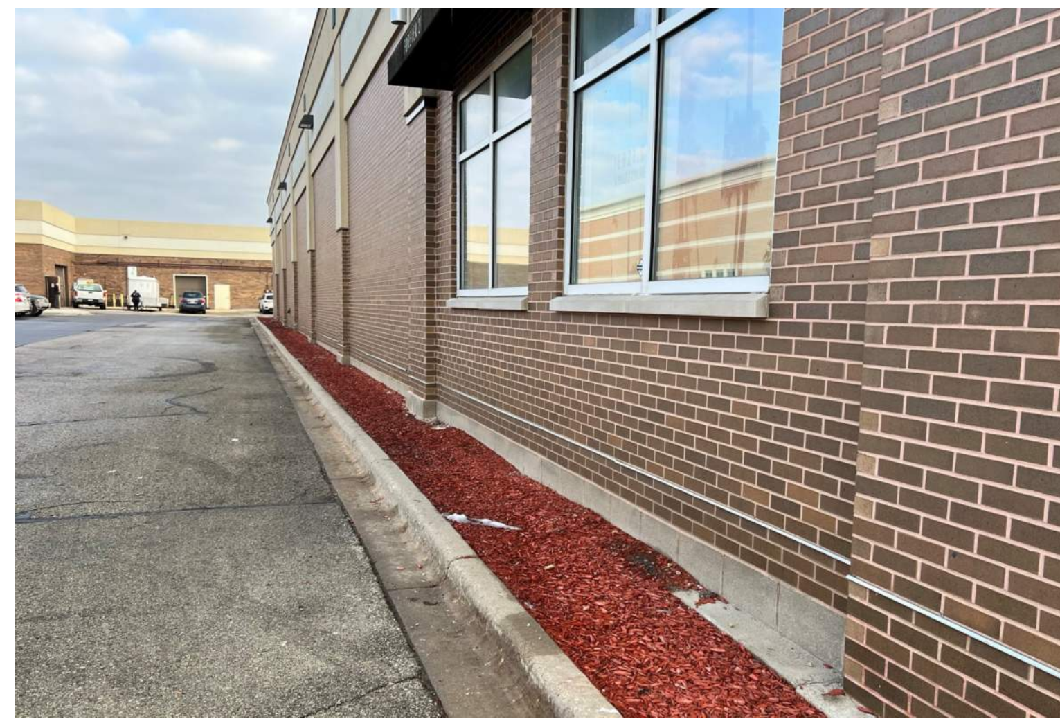
PLANET FITNESS NORTH EXTERIOR WALL
