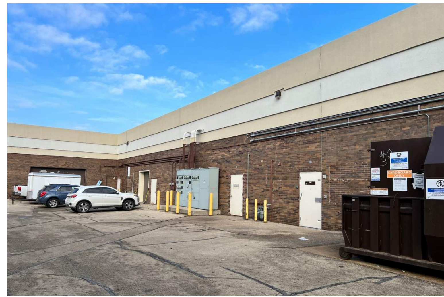
PLANET FITNESS NORTH EXTERIOR WALL
