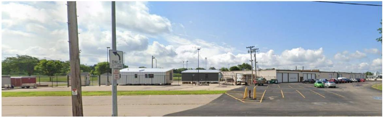
VIEW OF BUILDING B FROM COMMERCIAL AVE
