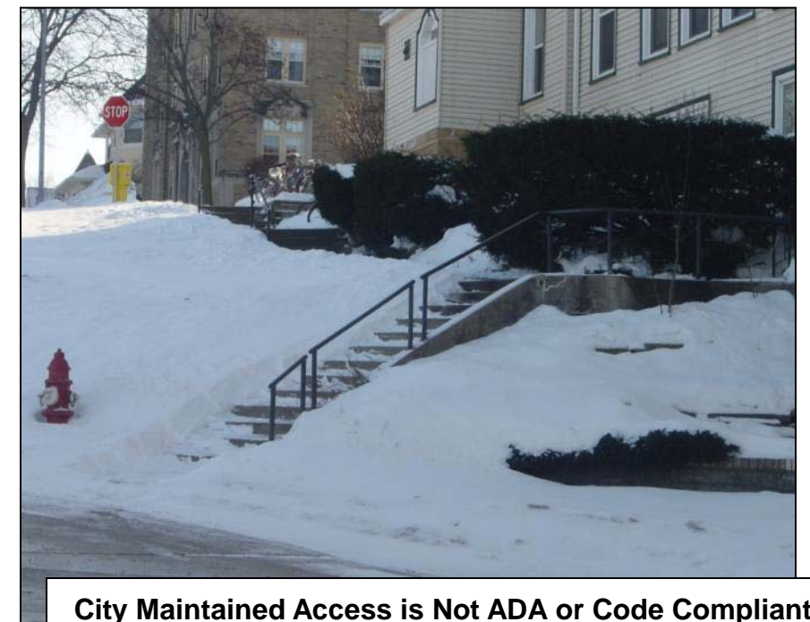
Slope is 10%, Maximum Allowed by Code is 5%
