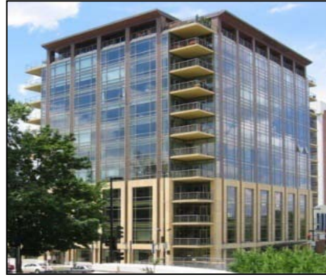
Condominium 100 Wisconsin Ave 9.7 FAR
