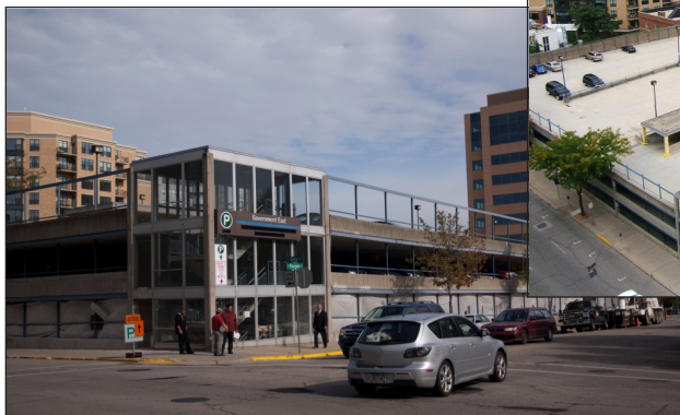
Government East Parking Garage, 2012
