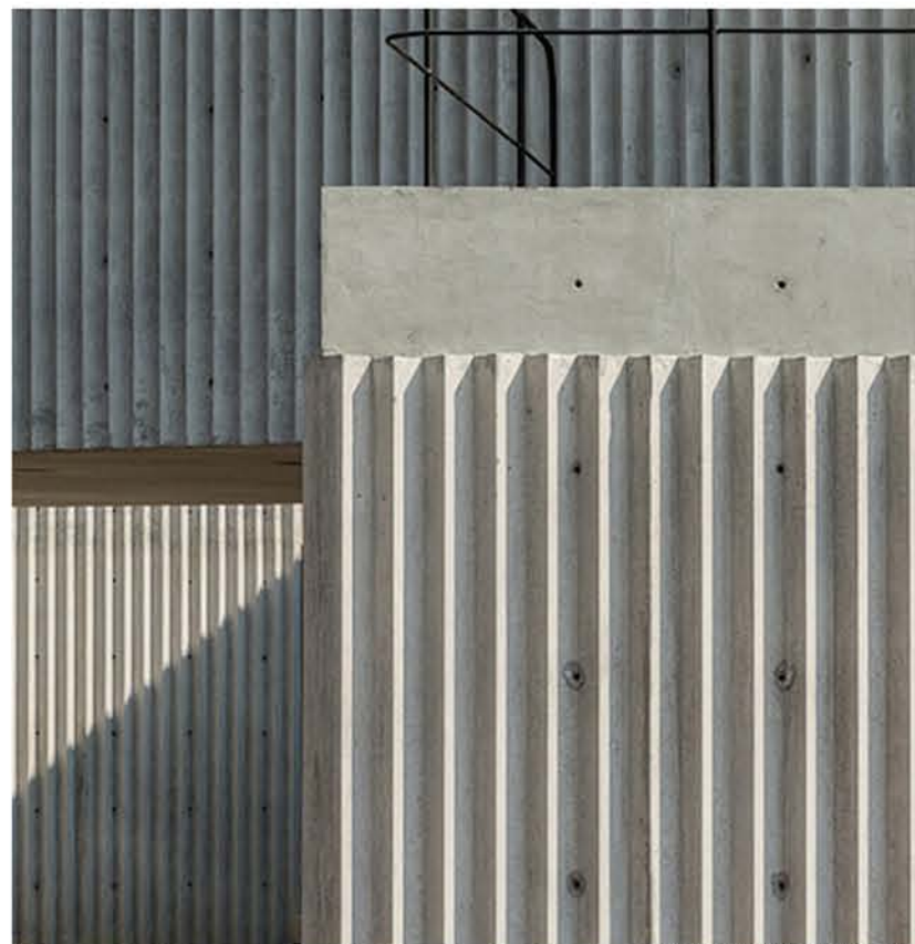
CORRUGATED CONCRETE FORMS housepstudiodope.com
