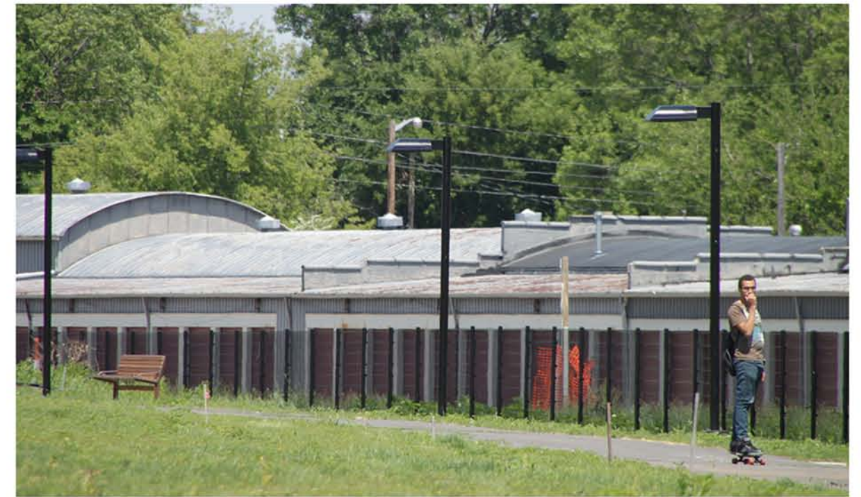
WELDED WIRE FENCE (MATCH CENTRAL PARK)
