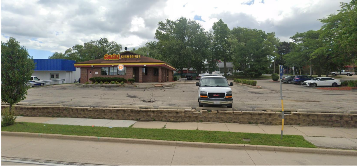
Figure 2: Existing Exterior view of project location (from E. Washington Ave)
