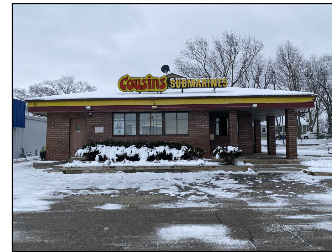
1 EXIST. NORTH PHOTO N.T.S.
