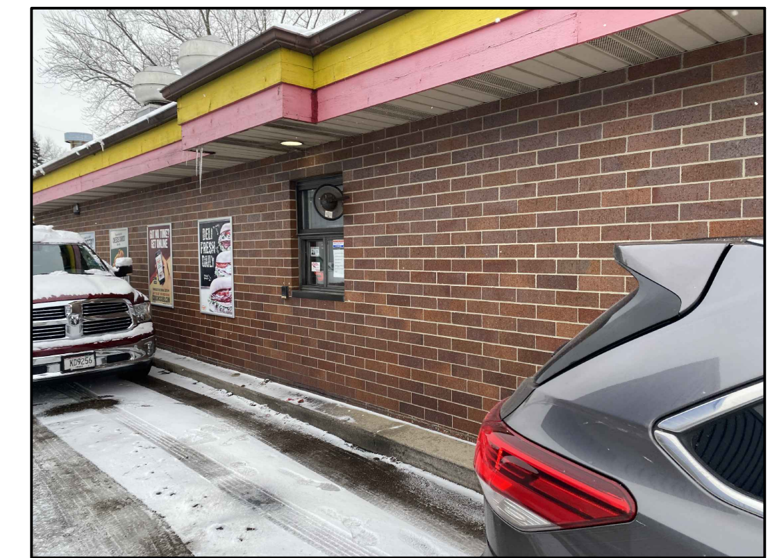
2 EXIST. EAST PHOTO N.T.S.
