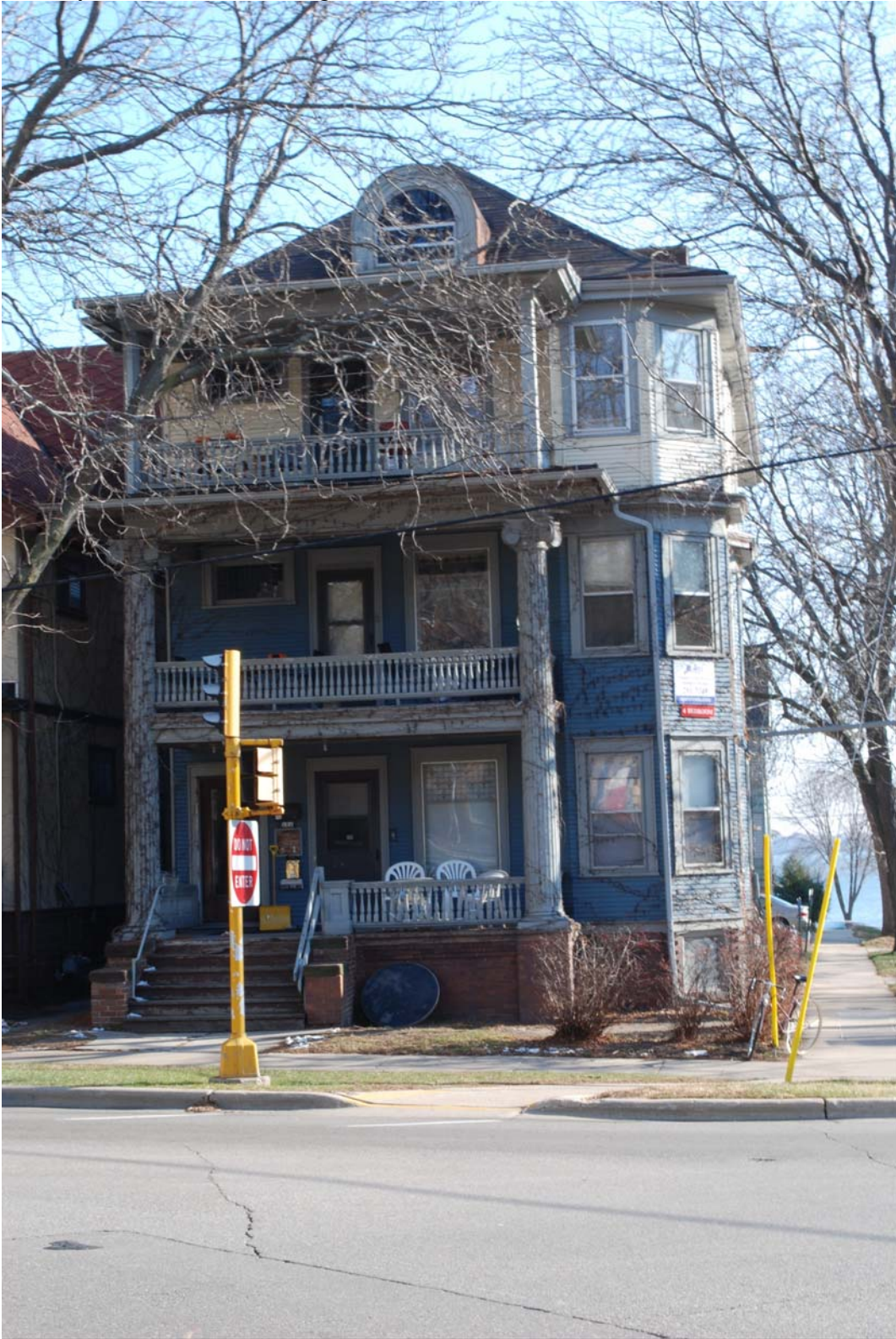
The Sayle Three-Flat Building, 153 West Wilson Street
