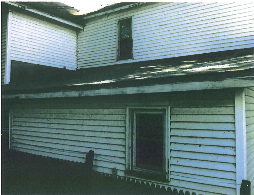
Rear addition/ Roof Area 3
