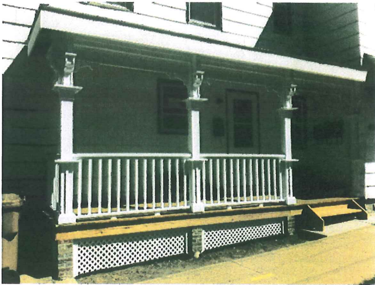
Front porch/Roof Area 1
