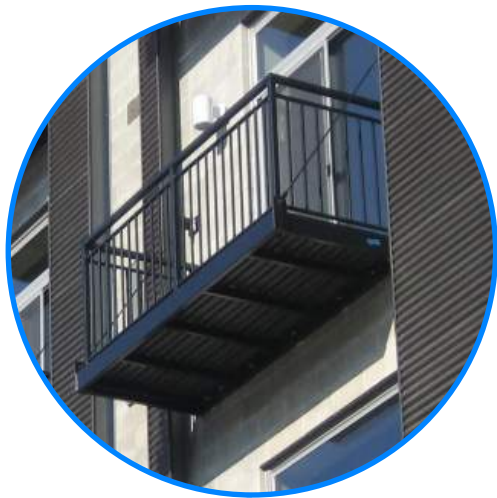
BLACK METAL BALCONIES, PICKETS, AND SUPPORTS
