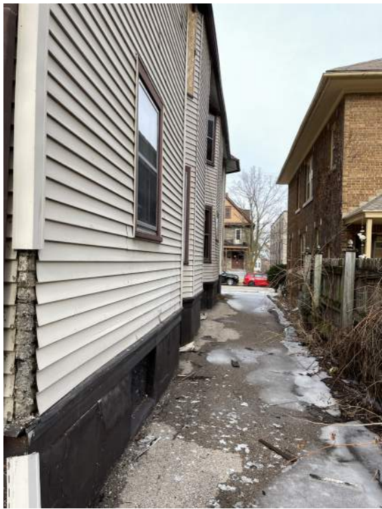
Driveway looking north
