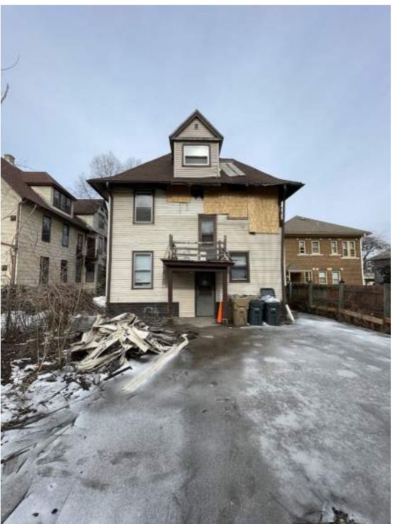
Parking area looking north
