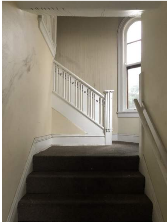
Stair up to second floor
