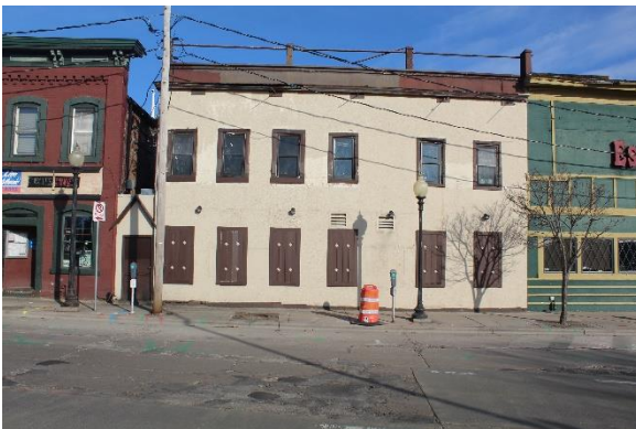
Front façade view of 510
