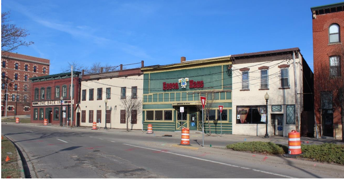
View of 506/608, 520, 524/526 and 518 East Wilson Street March 29, 2019.
