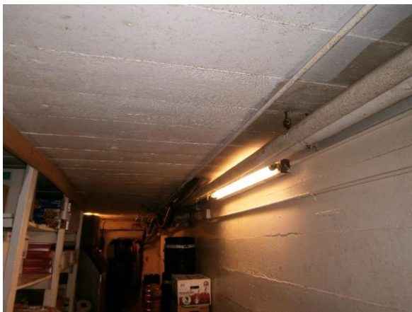
Concrete floor slab of first floor viewed from basement
