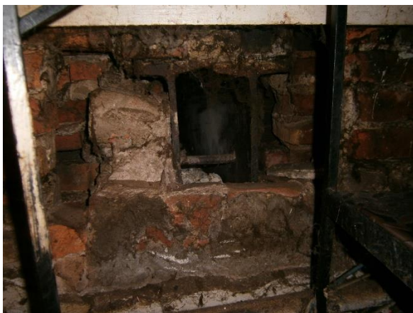
Steel beams supporting portions of second floor.
