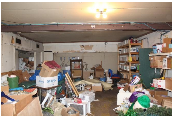
Second floor of 514/516
