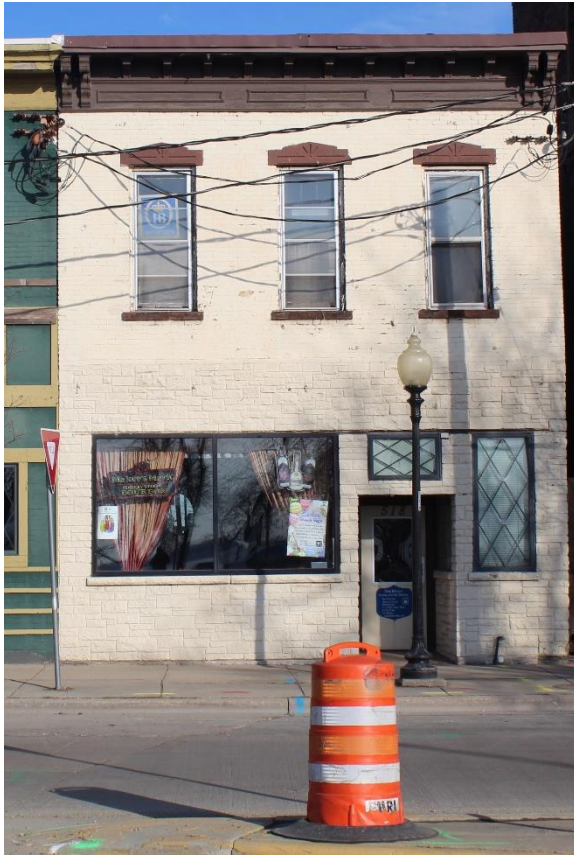
View of front façade of 118 East Wilson Street
