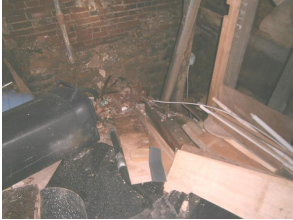
View of collapsed first floor at rear of building.
