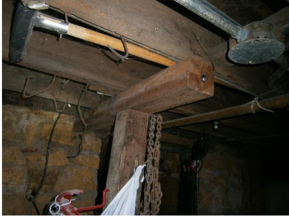
View of added support column and partial beam in basement.
