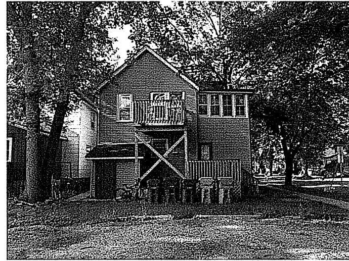
St. James Ct. Elevation (Rear)
