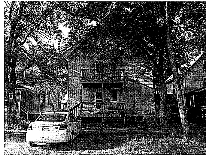
St. James Ct. Elevation (Rear)
