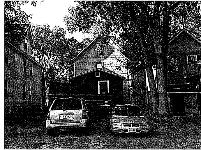
St. James Ct. Elevation (Rear)
