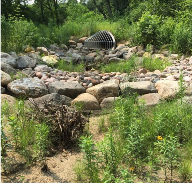
Improved Stormwater Management
